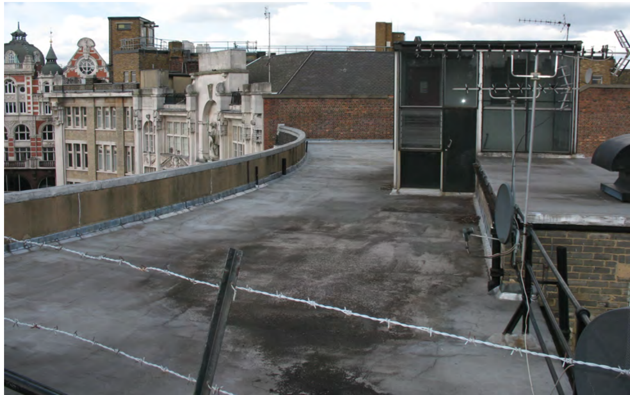
PH09 - The poor condition of the existing asphalt surface to the front flat roof
