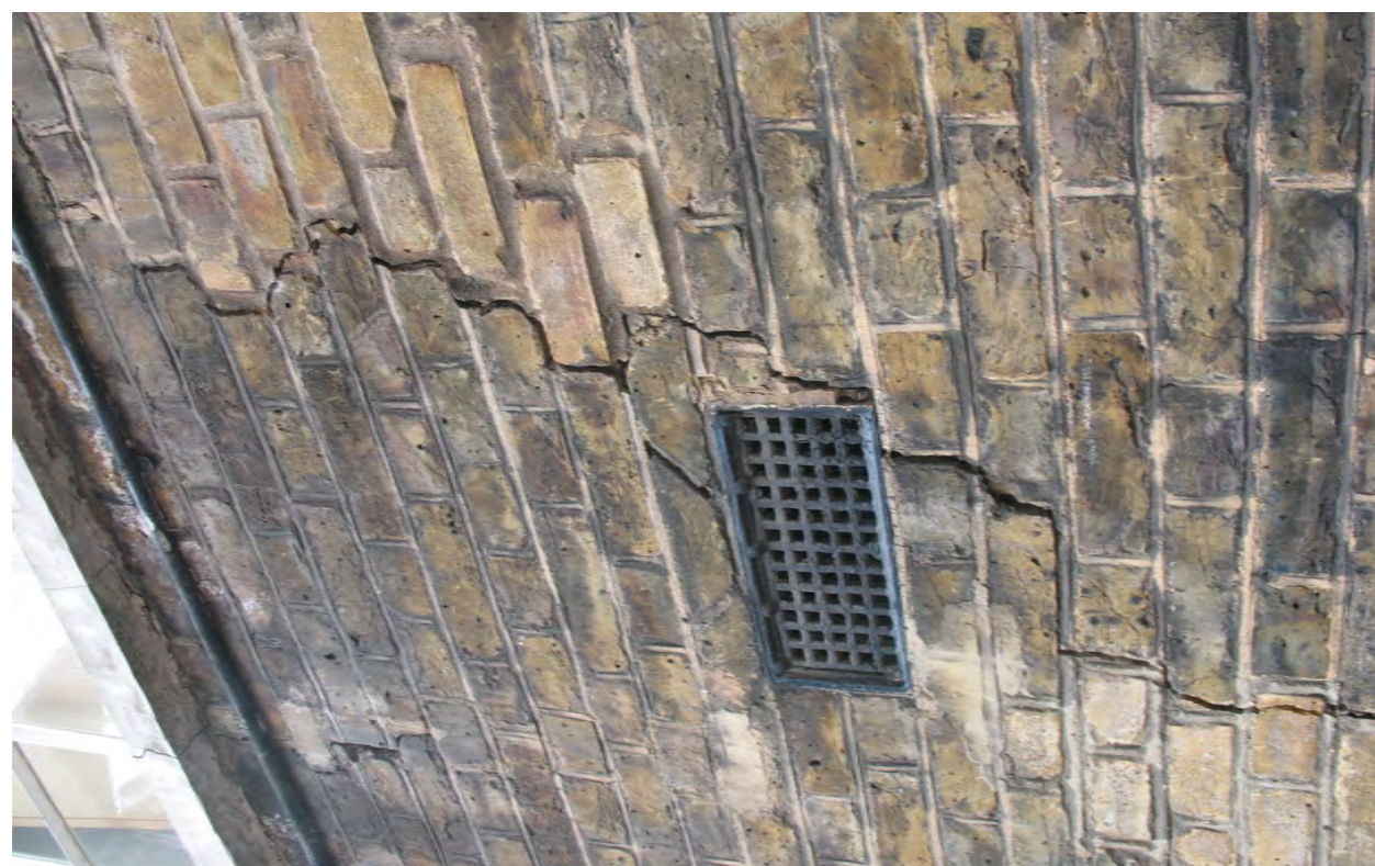
PH13 - The structural fracture to the brickwork to the side elevation
