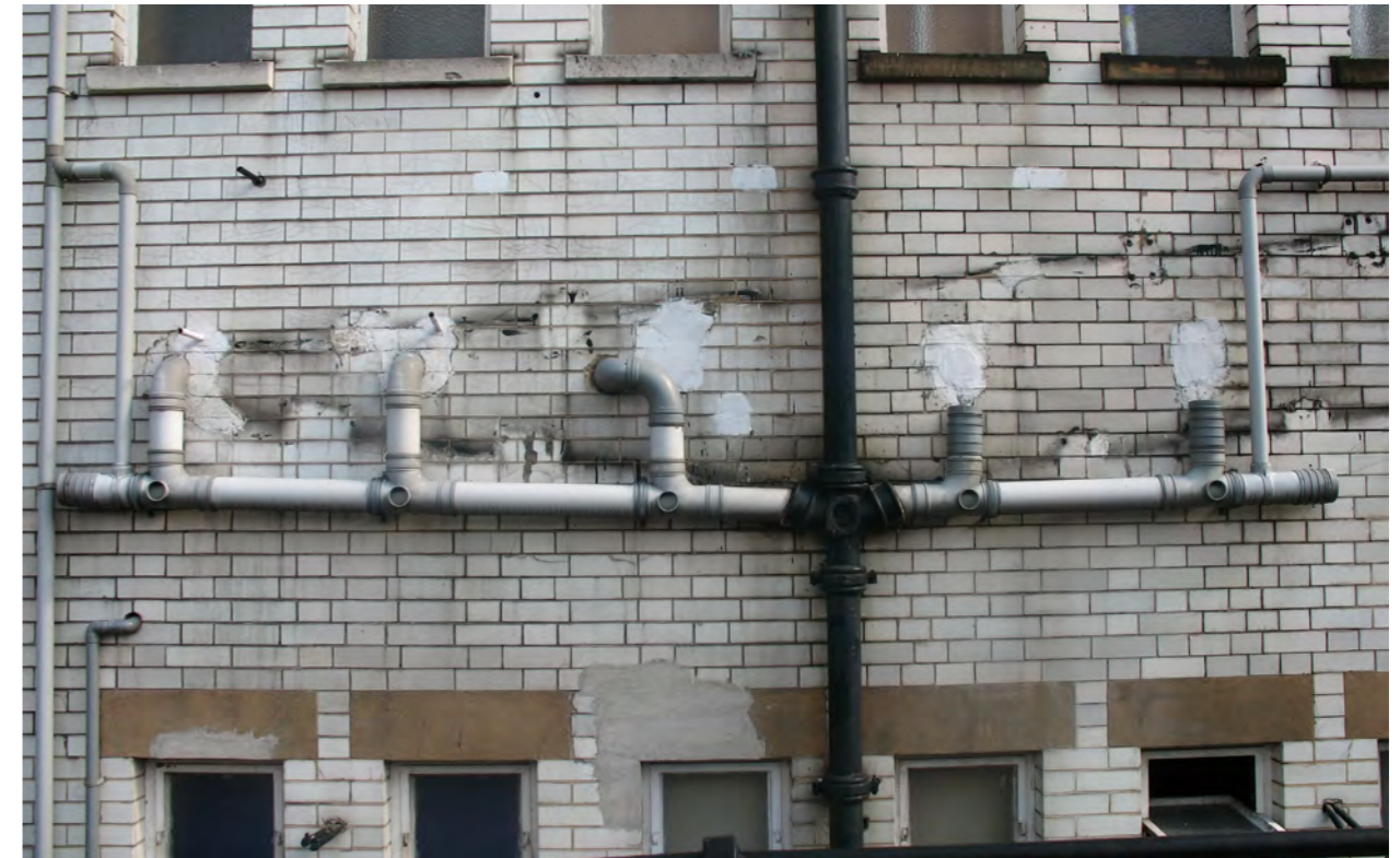
PH11 - The existing glazed faced brickwork to the rear wall of the front building
