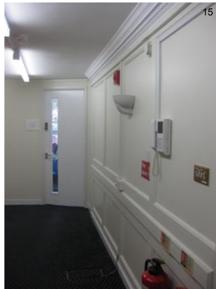
13 Typical cornice detail with partition junction
