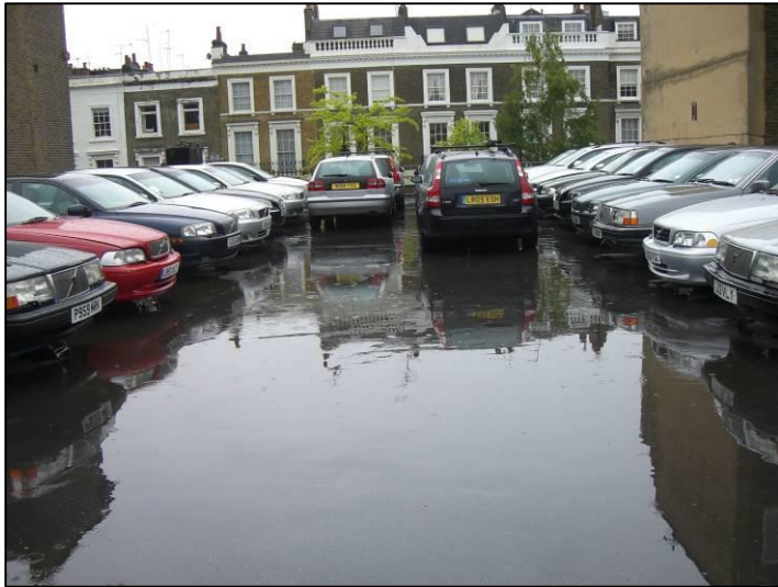
Photo 13. View of roof top car park
