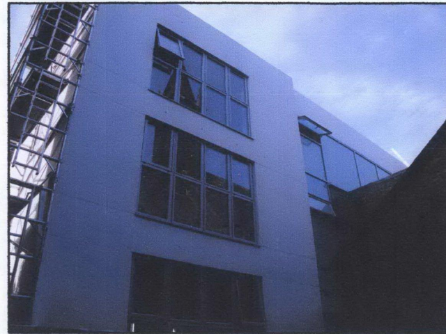
Side elevation view of curtain wall and render
