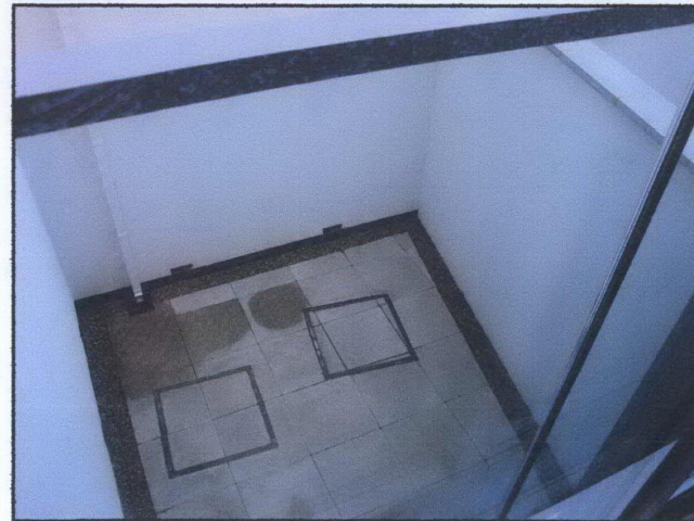
View of render and downpipe
