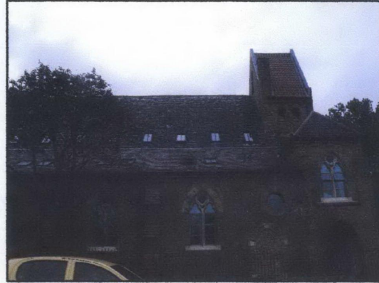
View of red roof tiles to the section of the roof fronting Loudoun Road. View of W20 steel section double glazed windows. View of the "Velux" Conservation style rooflights ref:GGLSD5N1 finished black as approved in PP dated 23/05/2007 your ref: 2007/1630/P and LBC dated 23/05/2007 your ref: 2007/1631/L.
