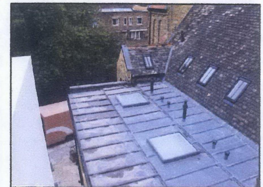
View of lead flat roof to the church conversion, "Timloc" low profile universal slate ventilator finished anthracite, "Duplus" flat roof deadlight ref: 8.3DL/AS size 1500 x 1500mm on plan and 200mm high finished grey. View of the "Velux" Conservation style rooflights ref:GGLSD5N1 finished black as approved in PP dated 23/05/2007 your ref: 2007/1630/P and LBC dated 23/05/2007 your ref: 2007/1631/L.
