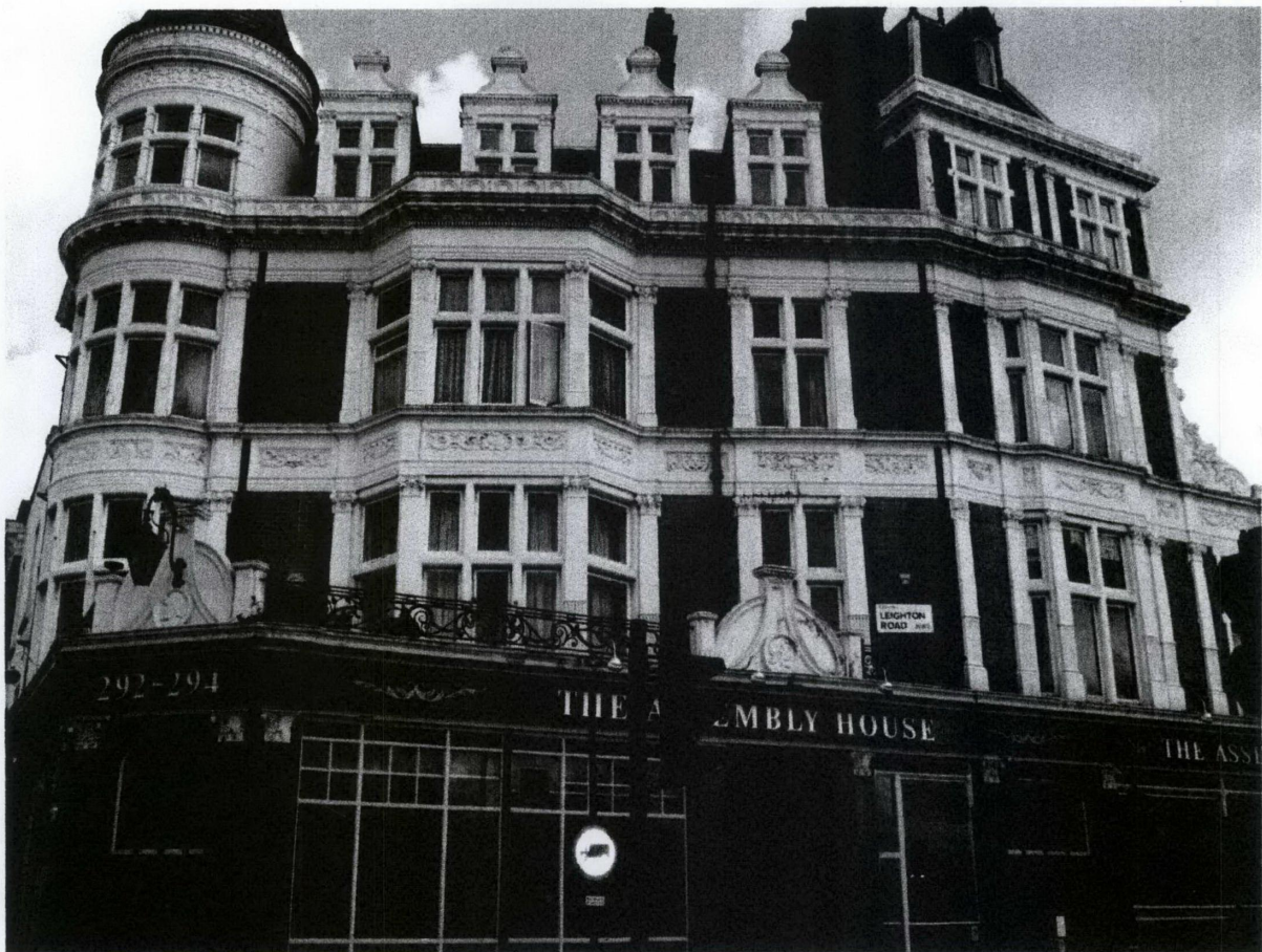
Photo #01 looking North East showing the front elevation from Kentish Town rail station.
