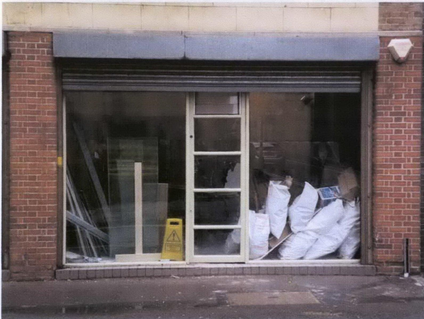
Ground Floor Shop Front showing Roller Shutters to be removed -Picture 3
