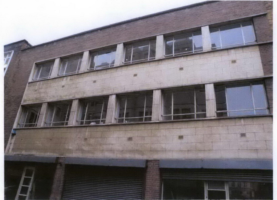
Shelton Street Windows to First and Second Floors - Picture 2
