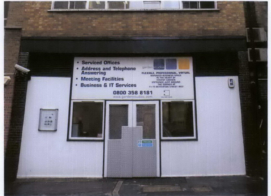
Entrance to 71-75 Shelton Street- Picture 6
