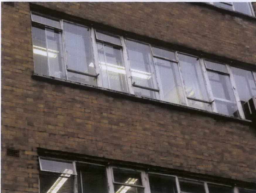
Window Detail to First, Second & Third floors of 71-75 -Picture 7
