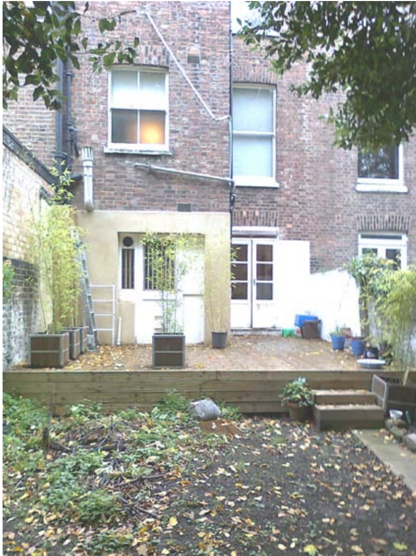
Existing rear elevation showing the rear extension of 5 Gladys Road which sets the height the proposed
