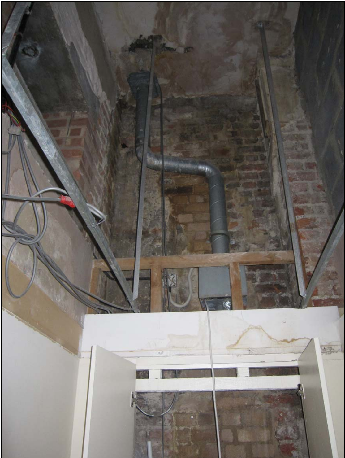
View of the lift shaft area, where one of the risers will be located. It can be seen that this area has been heavily altered in the past, including the erection of a modern block wall (right), new brick work and the insertion of modern services.
