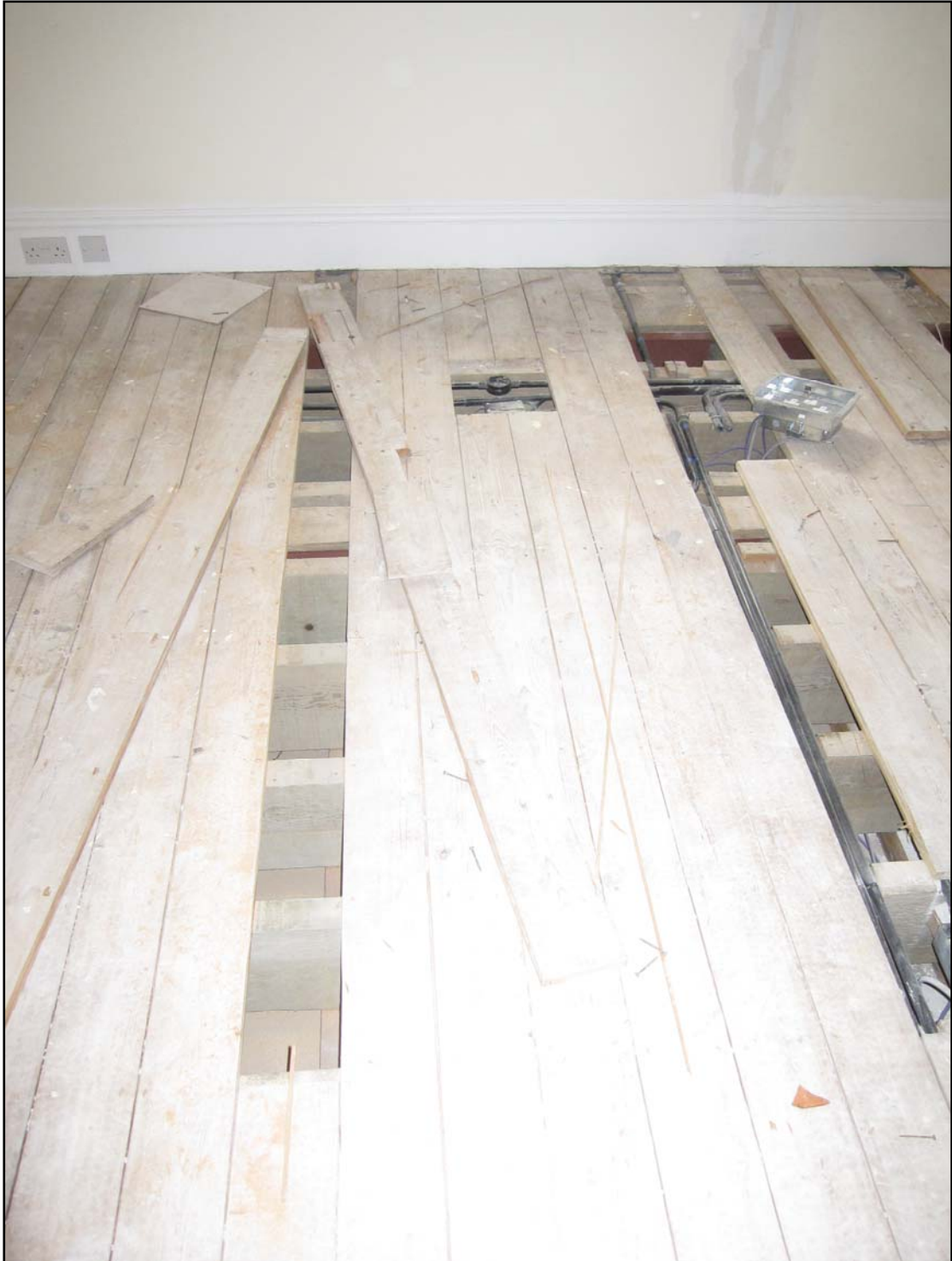
View of one of the 3 rd floor rooms with floor boards lifted. The modern floor boards and joists are clearly visible. Modern services have also been provided, note the electrical floor box in the top right. This is typical within the building.
