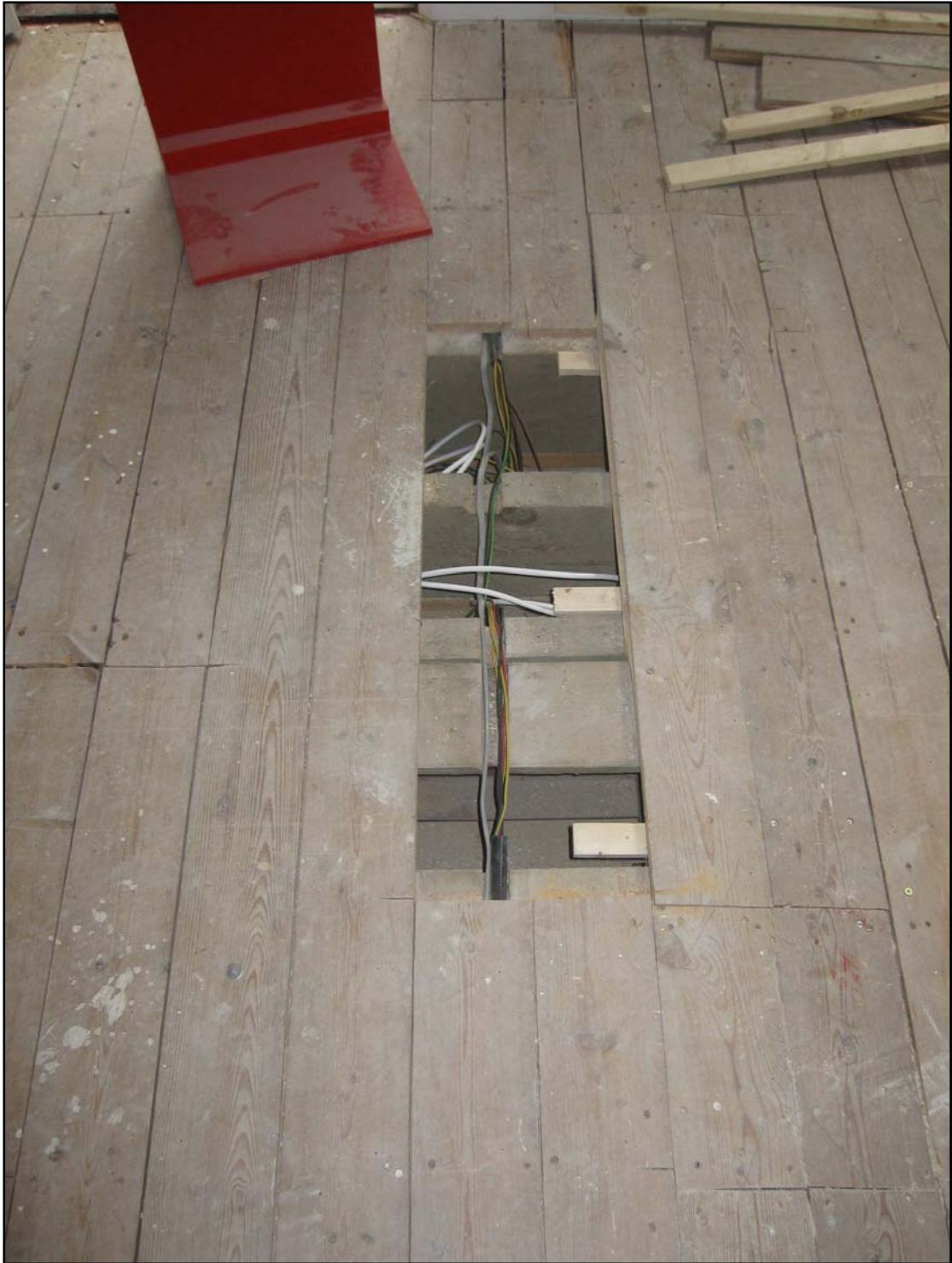
Modern data cabling running through existing notches in the joists. These existing notches can be largely re-used and old cable can also be removed.
