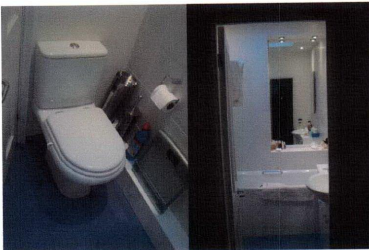
EXISTING BATHROOM AND SURROUNDING WALLS TO BE REMOVED
