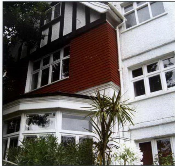
View of the existing site
