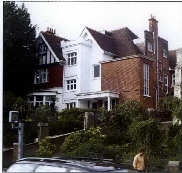
View of the existing site from Finchley Road
