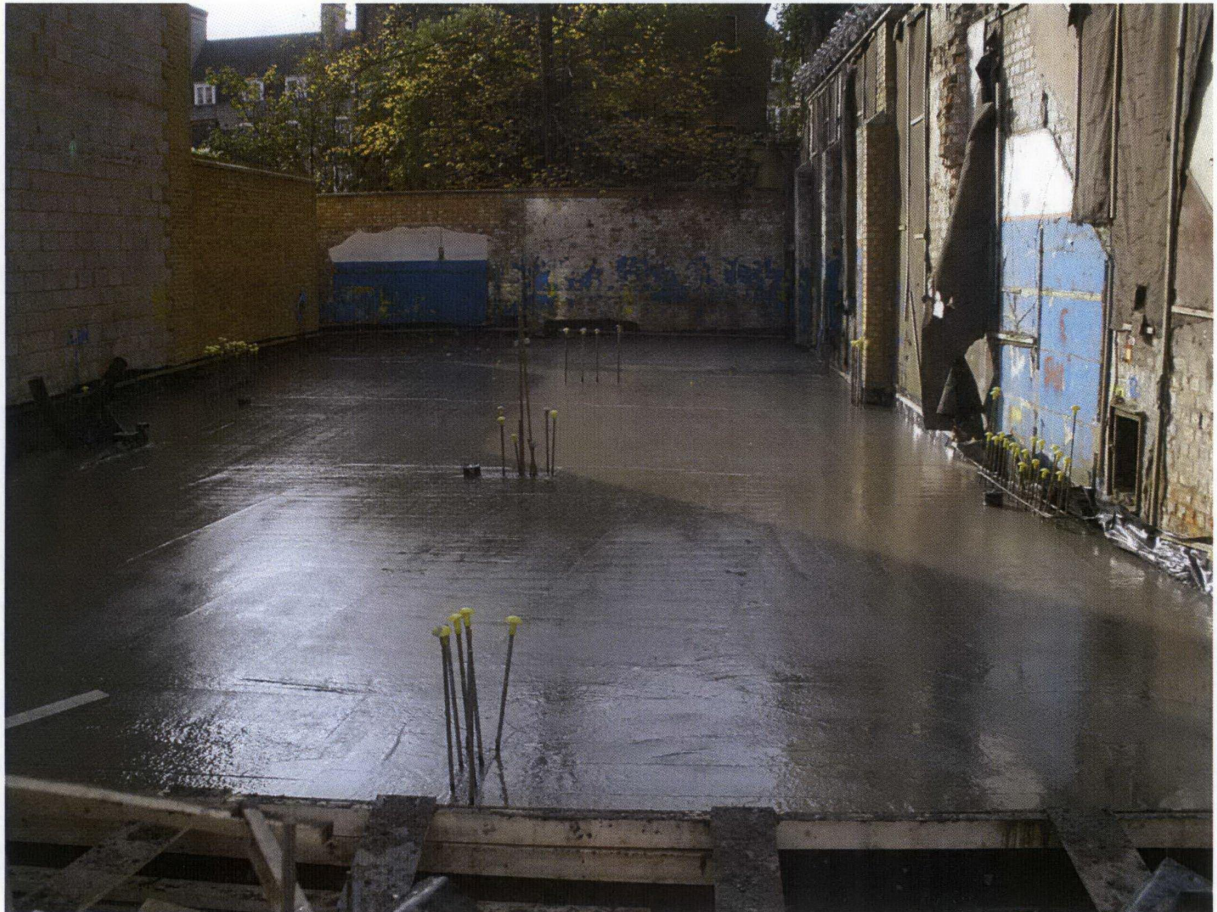
Ground slab covering the whole site
