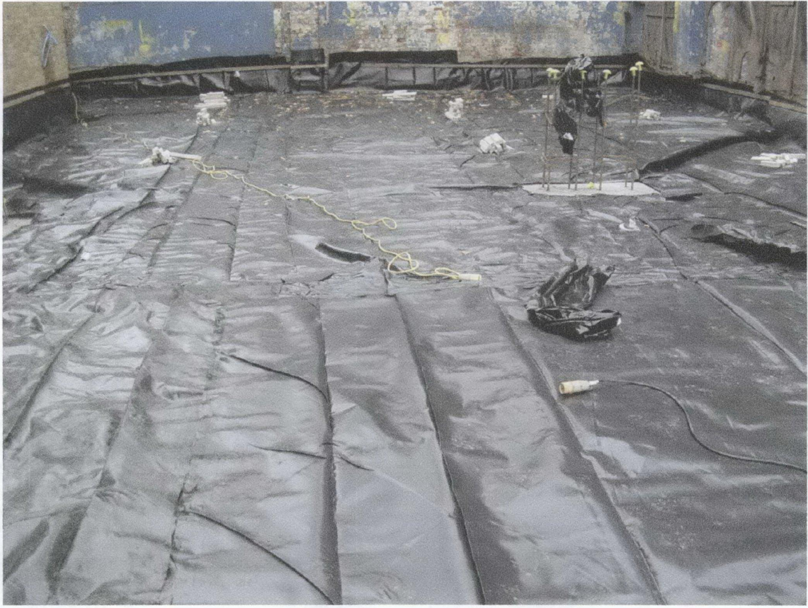
Laying out of Damp Proof Course
