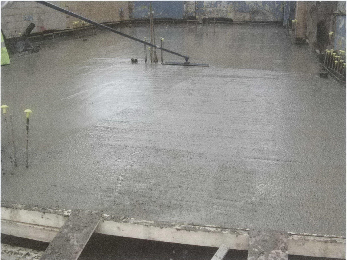
Pouring of the Concrete Slab
