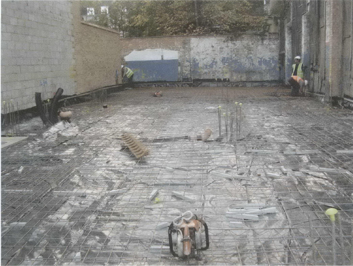
Laying out of the Concrete Reinforcement
