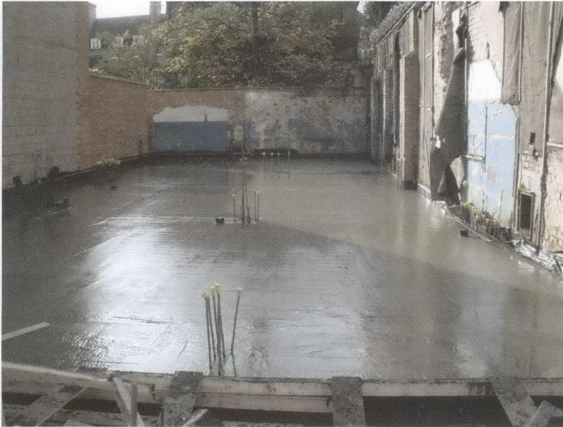
Finished Concrete Slab, thickness 275mm
