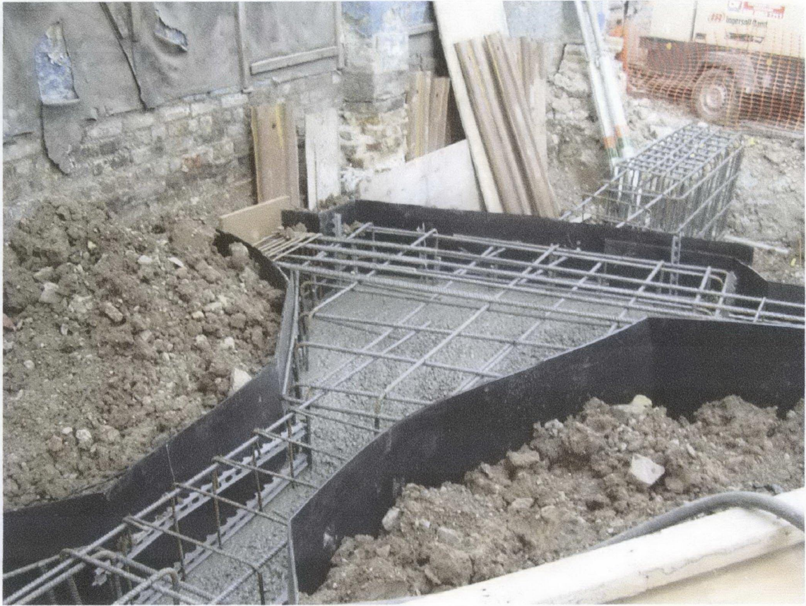
Construction of ground beams
