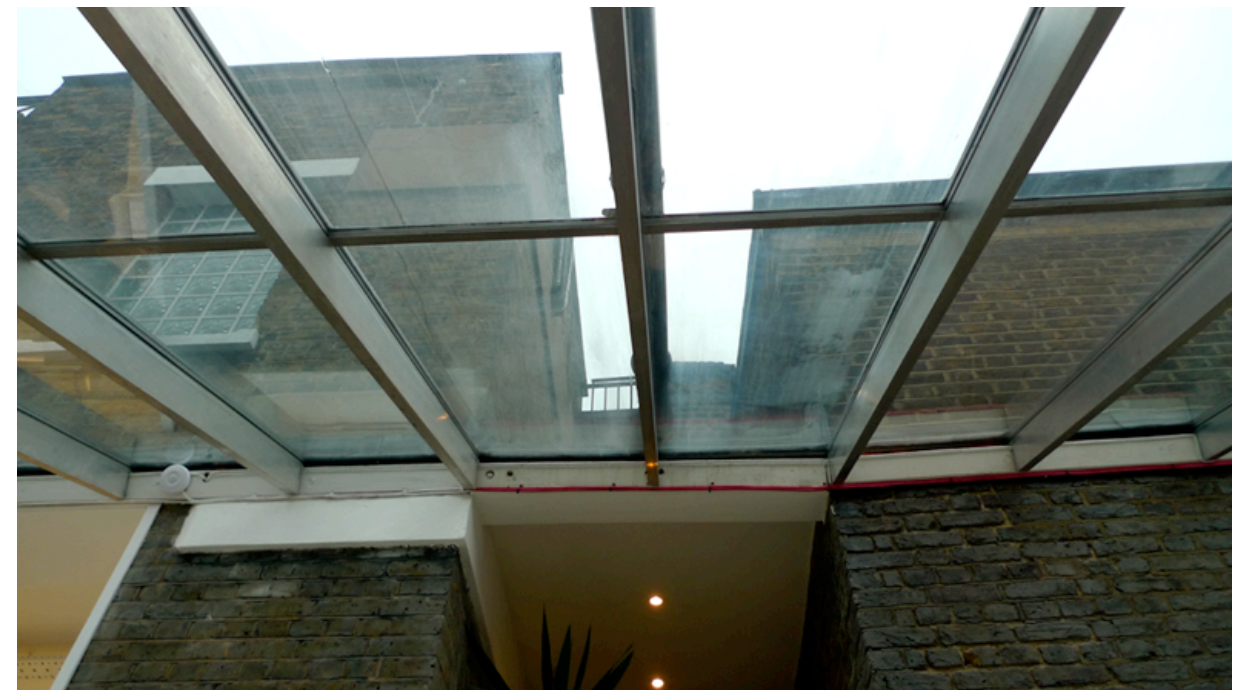
View of proposed lift location
