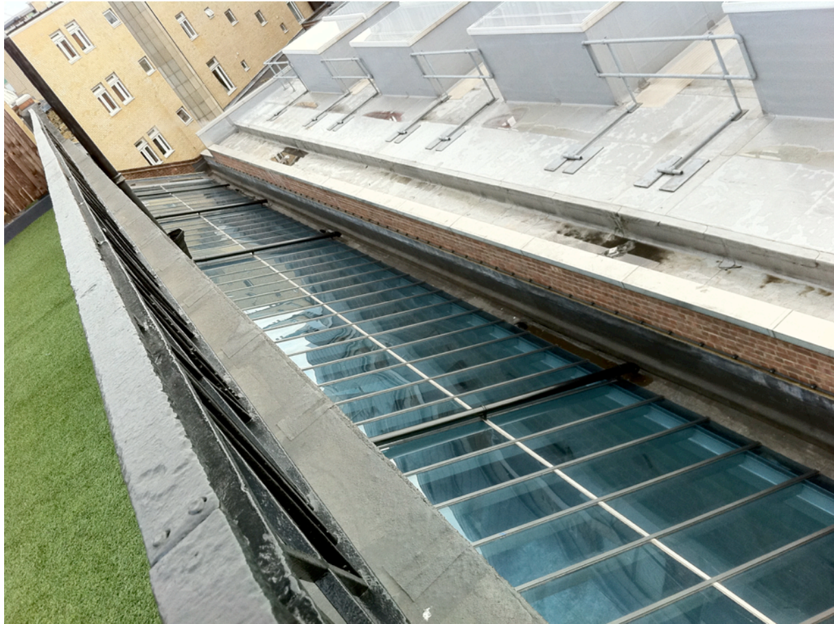
View from rear of roof terrace looking at lower glazed roof
