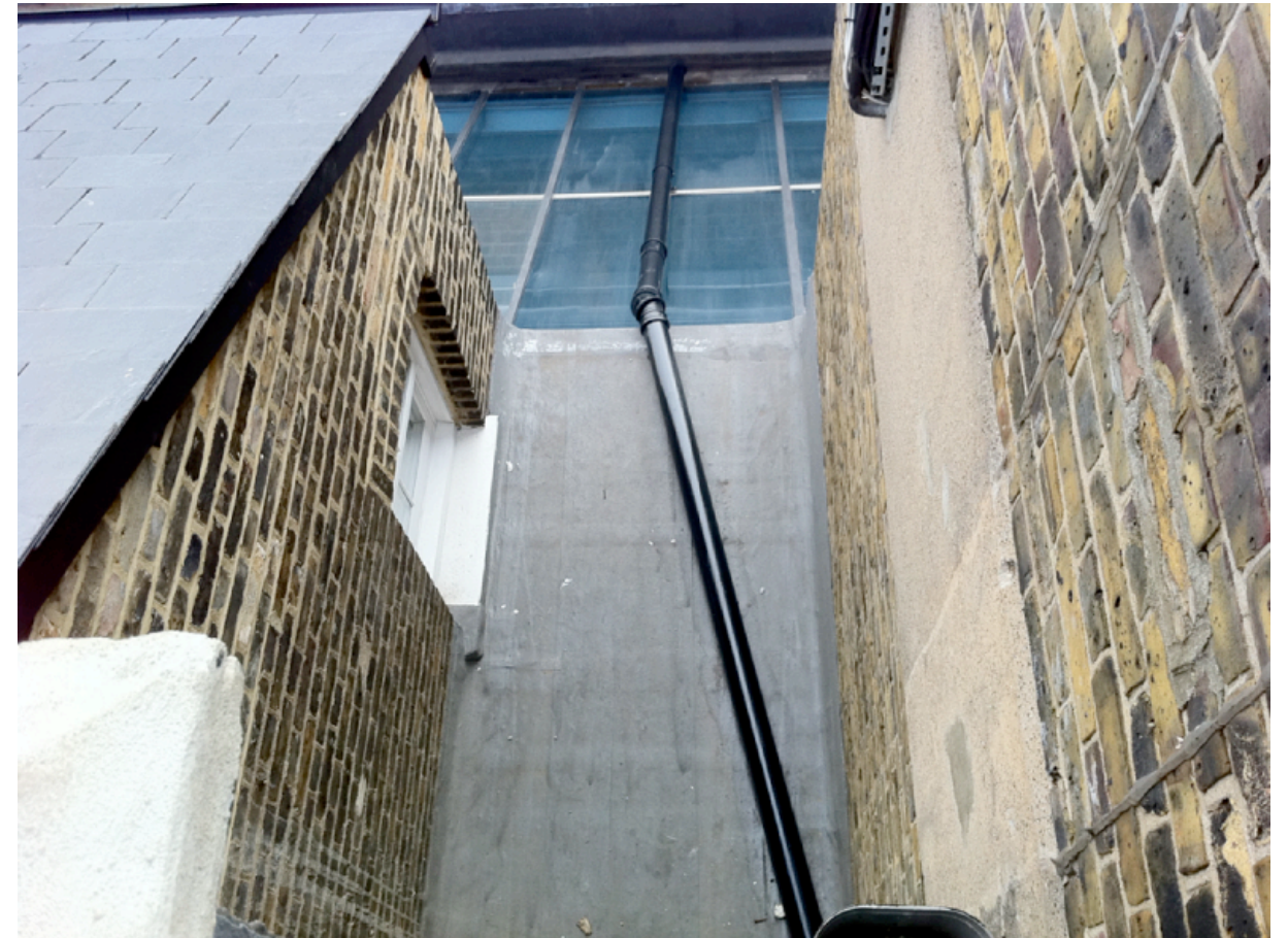
View of proposed lift location
