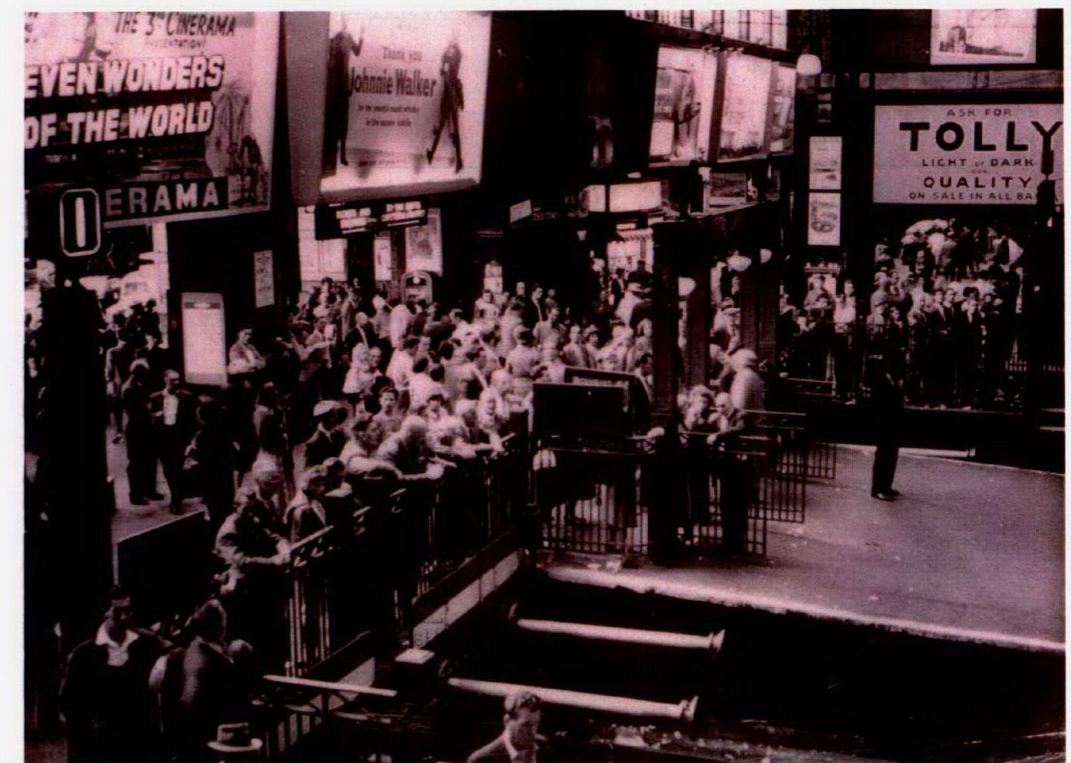
1950's view of head of platforms in the main shed
