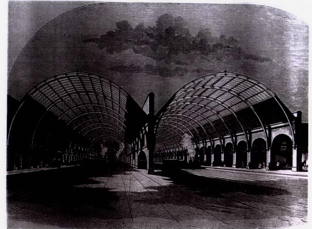
From The Builder , Vol X, No 504, 1851, showing the sheds with the front of the station removed and omitting the solid hipped slate roofs terminating the sheds at the north end.
