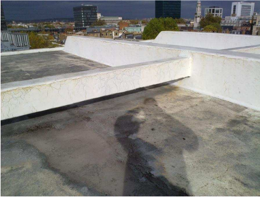
EXISTING UPSTAND BEAMS
