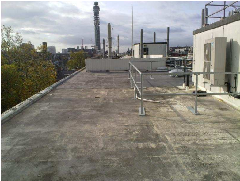
GENERAL VIEW OF EXISTING ROOF
