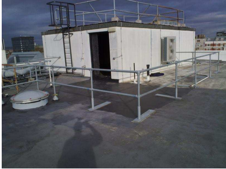
EXISTING MASONRY ENCLOSURE WALL AND SAFETY HANDRAIL
