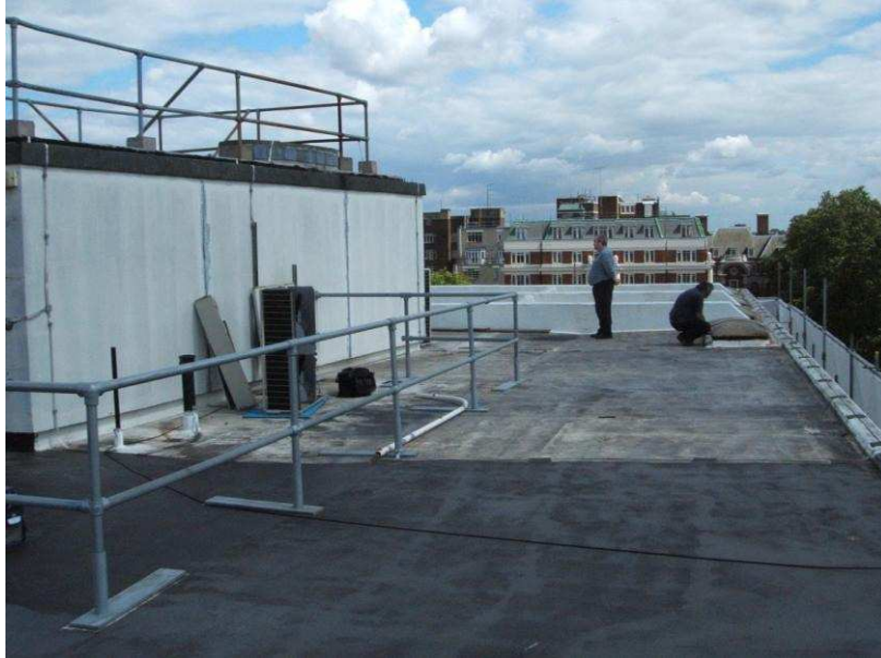
GENERAL VIEW OF EXISTING ROOF
