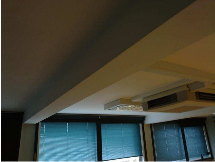
EXISTING DOWNSTAND BEAM BELOW ROOF SLAB
