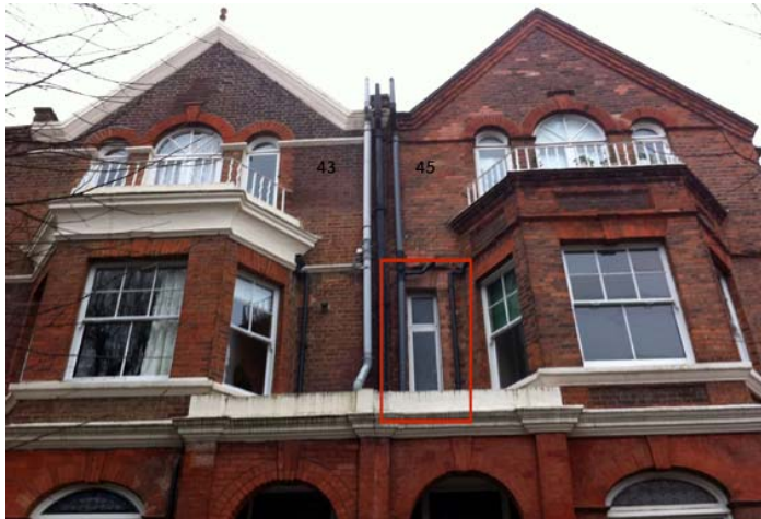
Existing window at no45 First floor level
