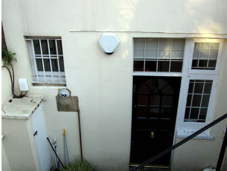
Existing Door and windows at LGF level light well.
