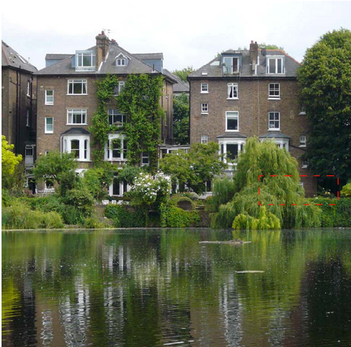
View from the other side of Hampstead Heath Pond No 2. The application site is the right hand lower ground floor, almost completely hidden by the large willow tree.
