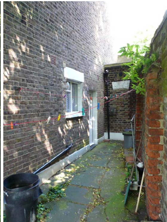
Currently redundant yard to the side of the property
