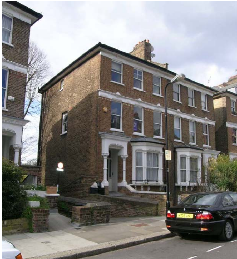
Front view of 96 South Hill Park
