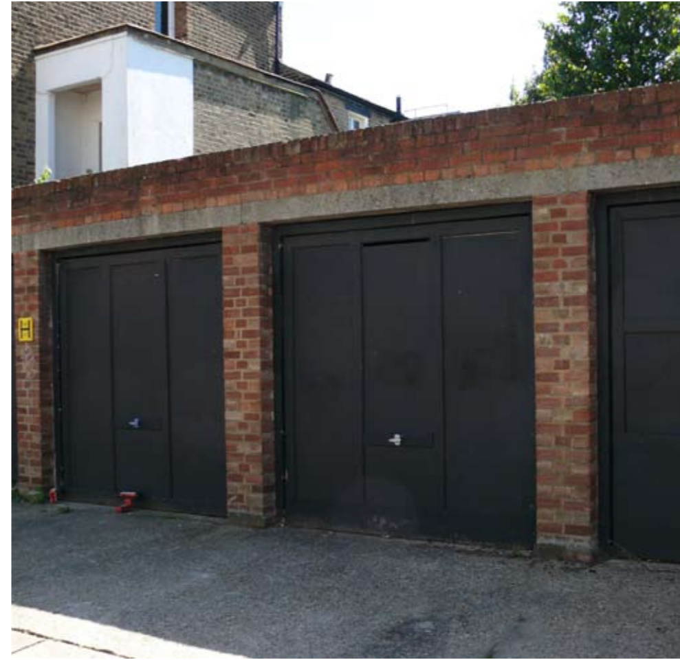
Simple red bricked garages.
