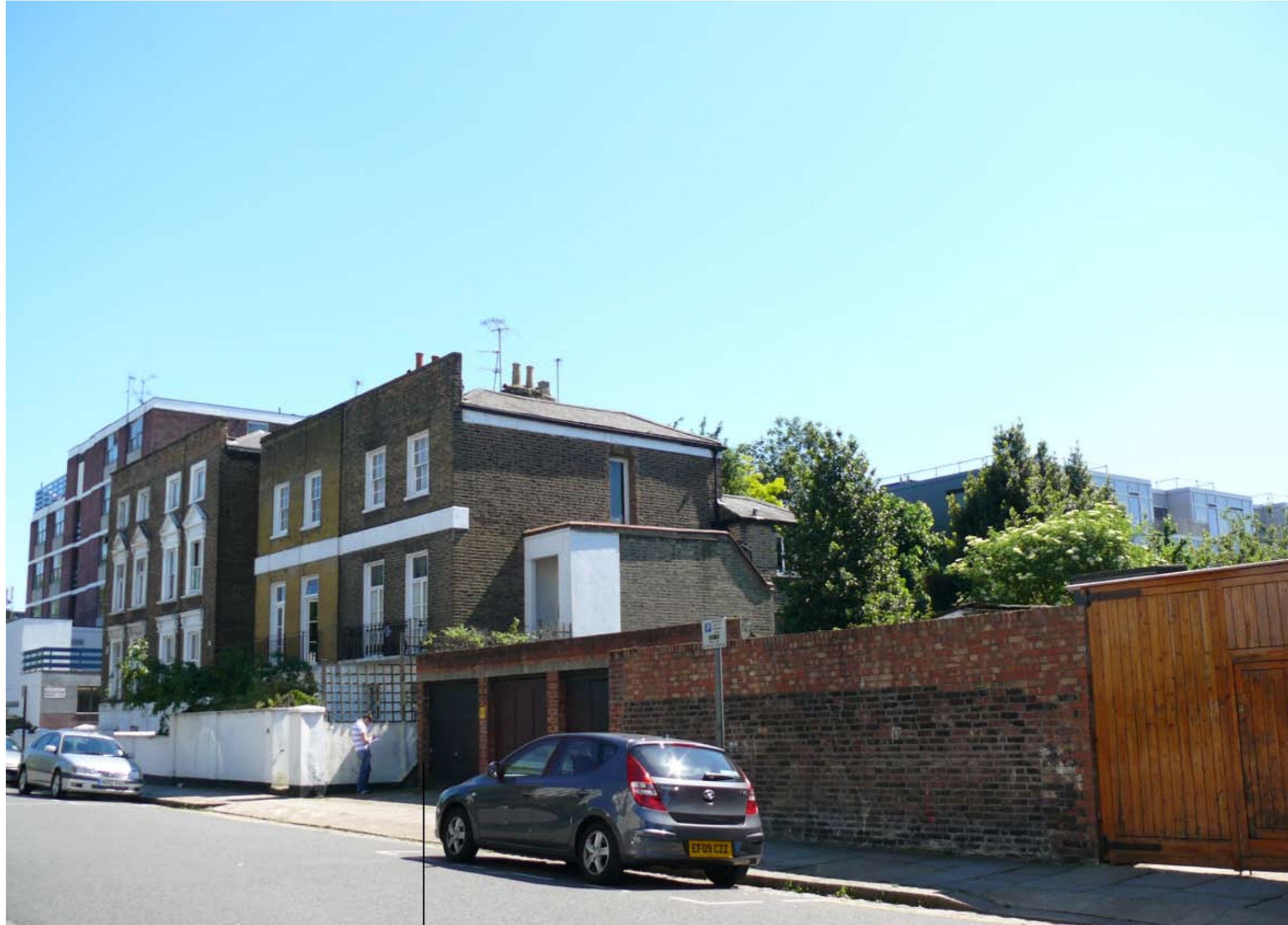
Poor quality garages facing Rochester Road
