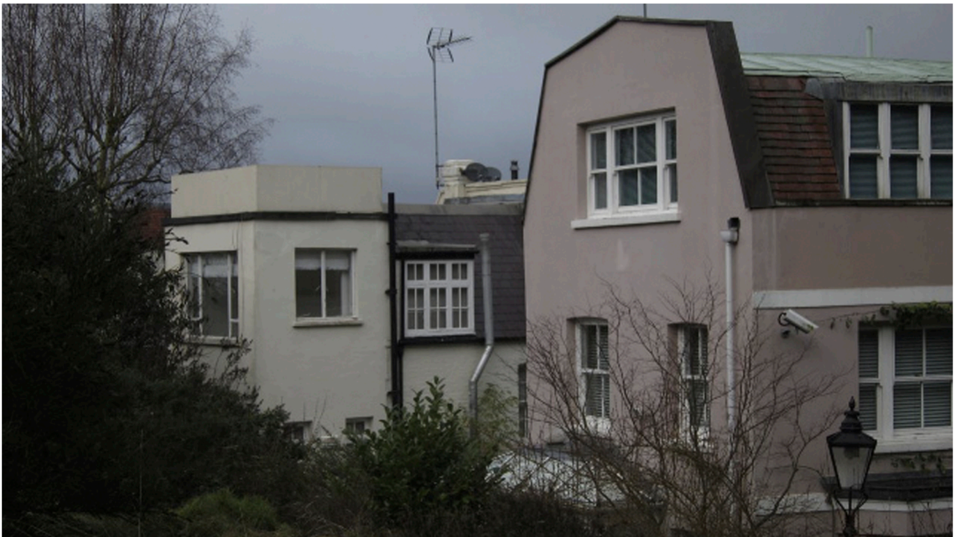
Detailed view from the Heath, showing the side and rear elevation to the existing extension to 1 Sandy Road (on the left). The view shows the existing windows that are proposed to be removed, and replaced with painted softwood double glazed windows. The rear, smaller window, is also proposed to have its cill lowered to come into line with the cill of the side window.
