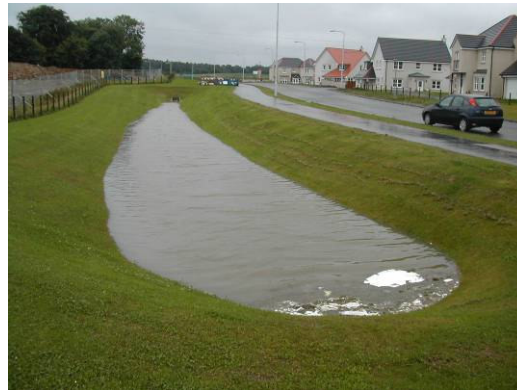
Figure 12 – Illustration of a detention basin following a period of heavy rain
