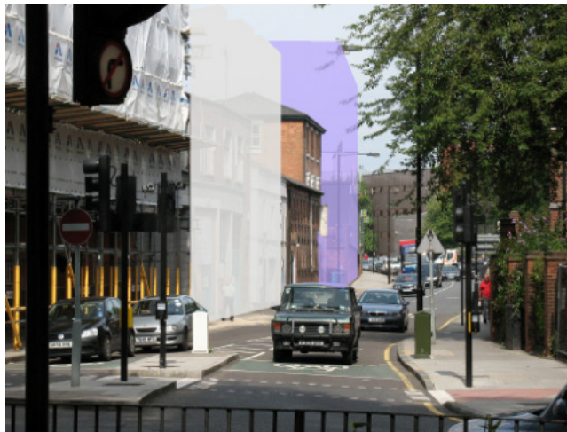
Fig - 5.6.2 - Critical View from Goldington Square (The white space is a neighbouring development)
