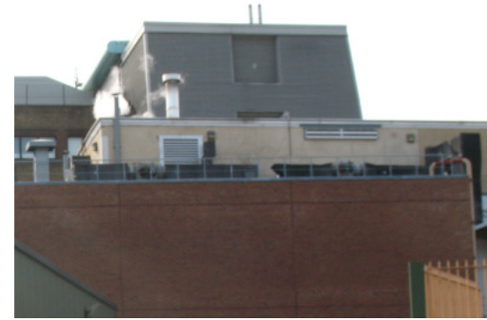
Fig - 5.8.4 - View through to the Rear of The Site
