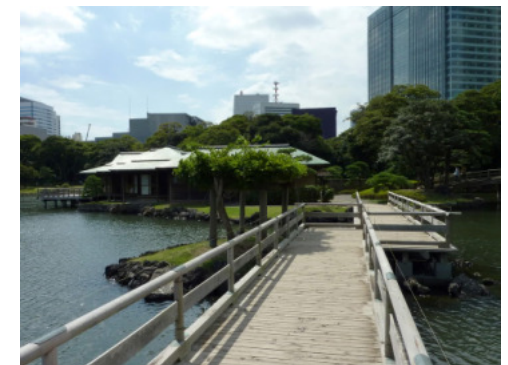
Fig - 4.4.2.2 - Stepped Bridges
