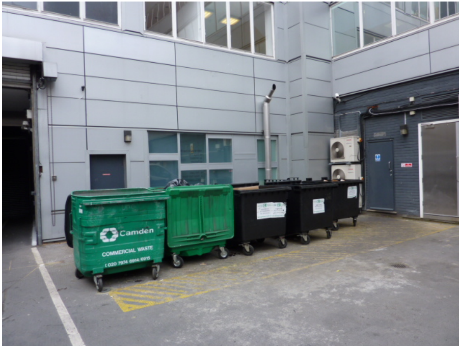
Image 12. Rear of Ground Floor Shops
