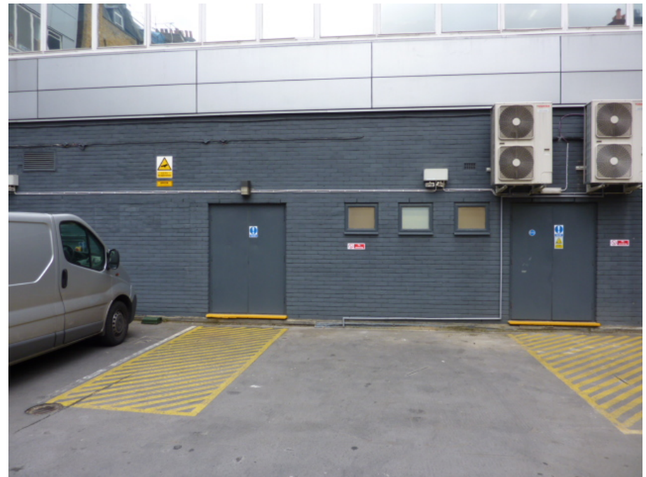
Image 11. Vehicular Entrance off Greys Inn Road
