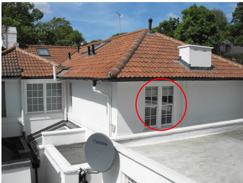
Figure 1 Window at 98 Frognal facing the existing garage
