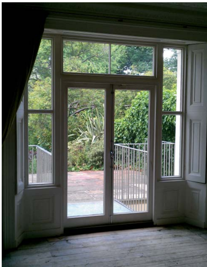
WINDOW WG4- Rear single glazed. Original frame and Modern door, modern blocked sashes
