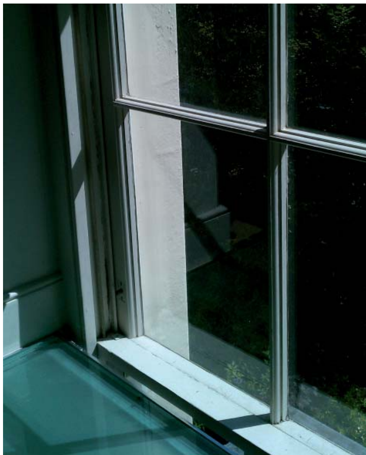
WINDOW W1.2- Front single glazed modern stair well windows
