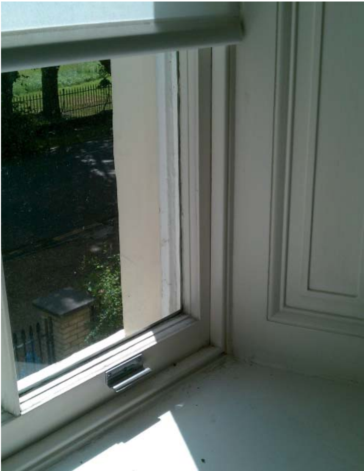
WINDOW W1.1- Front original single glazed sashes
