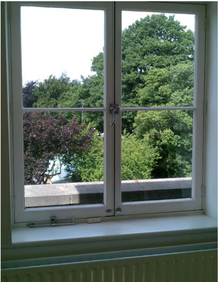
WINDOW W3.4- Rear modern single glazed casement window to dormer from 2000
