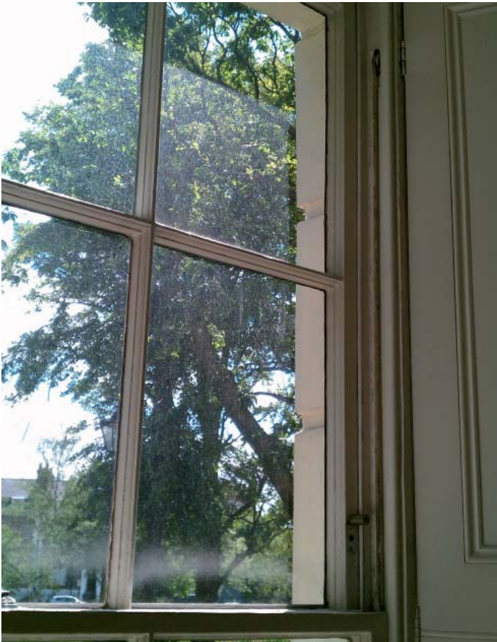
WINDOW WG.1_ Original single glazed to front
