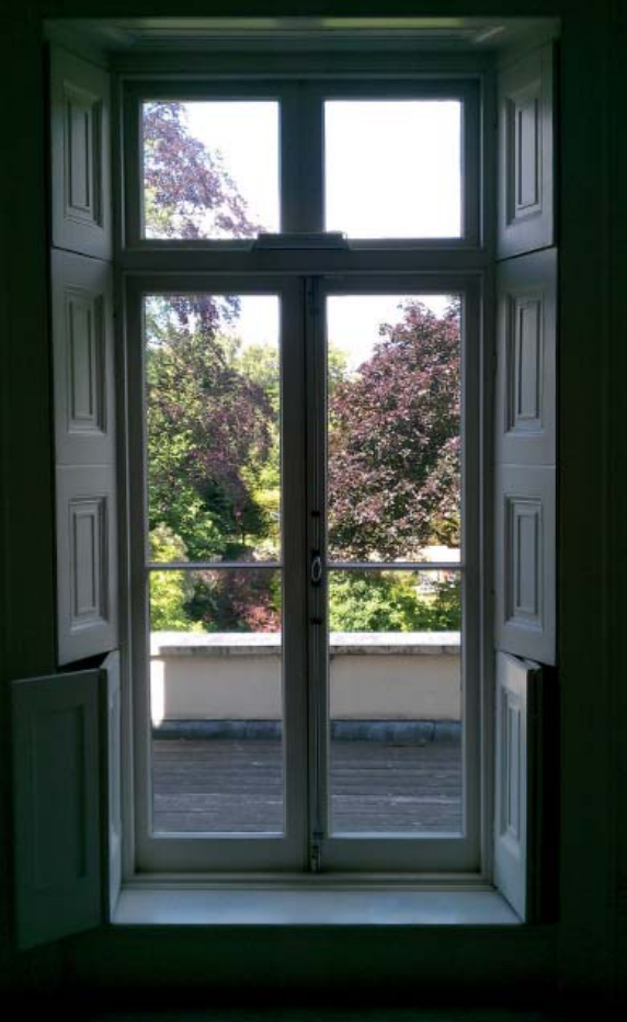
WINDOW W1.5 - Rear modern single glazed french doors 2001. Original frames.
