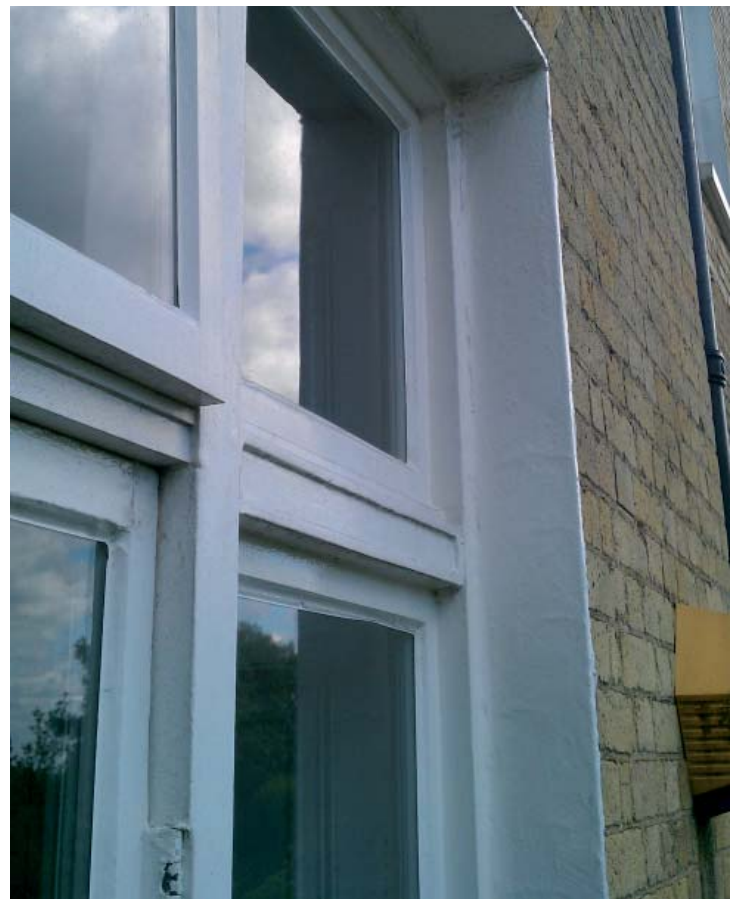
WINDOW W1.4- Rear single glazed. Original frame and original door door, modern flanking fixed panels
