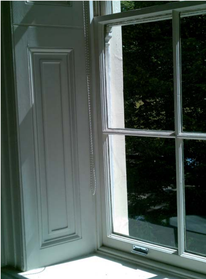
WINDOW W1.1- Front original single glazed sashes
