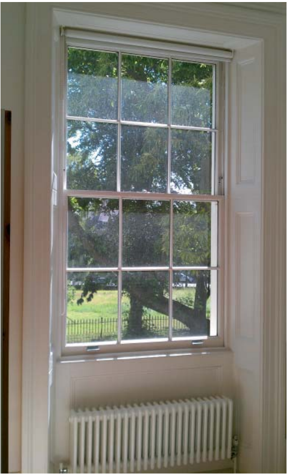
WINDOW W1.3- Front modern double glazed sash
