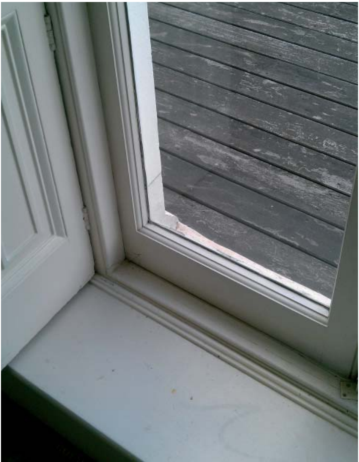
WINDOW W1.5 - Rear modern single glazed french doors 2001. Original frames.
