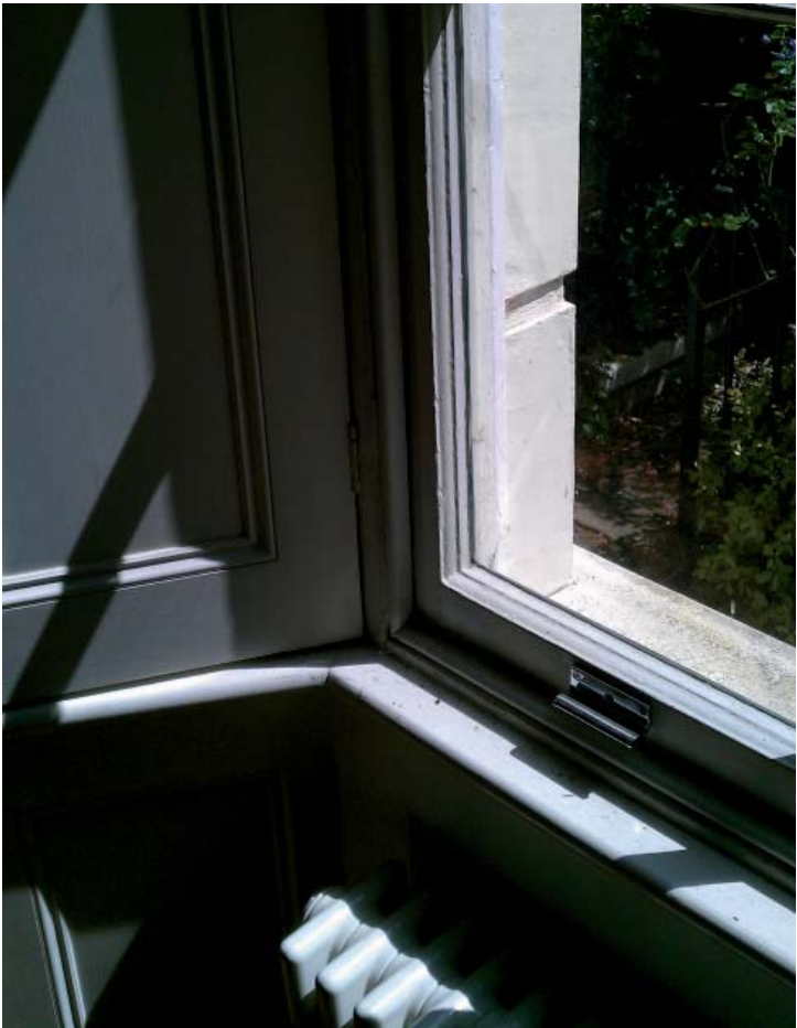
WINDOW WG.1_ Original single glazed to front
