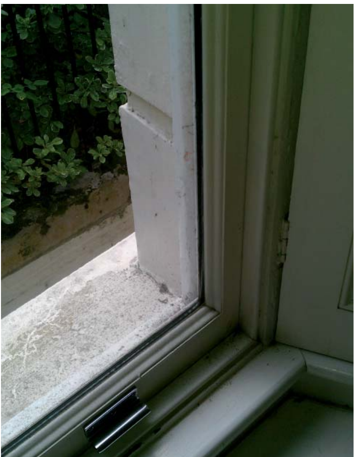
WINDOW WG.3 _Modern double glazed to front kitchen
