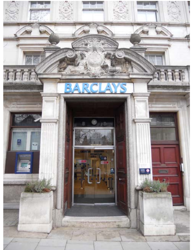
28 Hampstead High Street – Entrance
