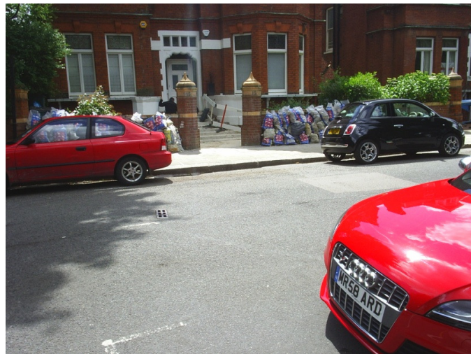
Figure 2 Lowest Point in Road with 12 Lyndhurst Gardens
