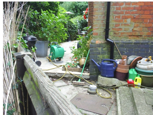
Figure 4 Side Terrace of No. 18 with Downpipe
