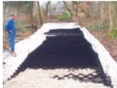
Installation of the CellWeb™ system.
