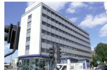
British Transport Building Adjacent to the site as height reference
