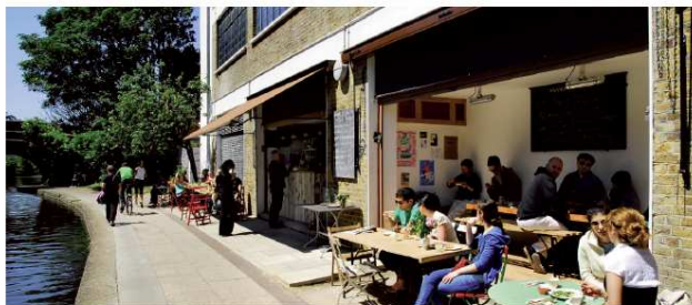
The Refurbished Bankstock Buildings, N1
