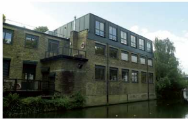
Canal Side Brick Converted Warehouse
