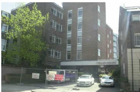
Photograph showing the entrance to Twyman House on Bonny Street
