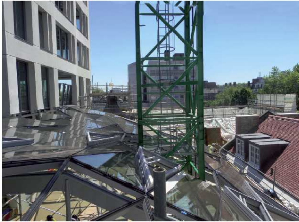
Unison Headquarters, Camden, London
