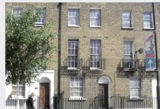
Residential 19th Century Terrace Typical of Camden Town
