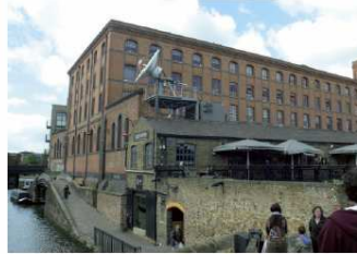
Canal Side Brick Converted Warehouse
