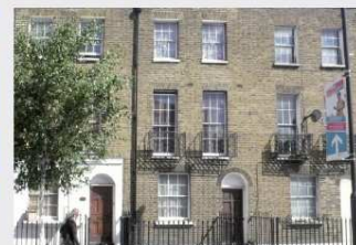
Residential 19th Century Terrace Typical of Camden Town
