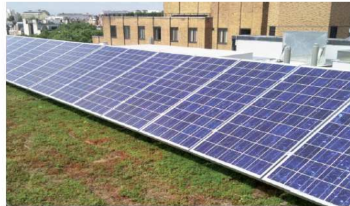
Green Roof and PVs at 1 Grafton Street, London.
