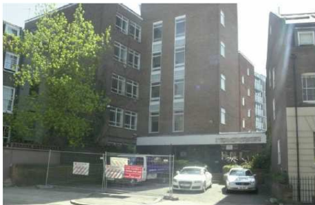
Photograph showing the entrance to Twyman House on Bonny Street
