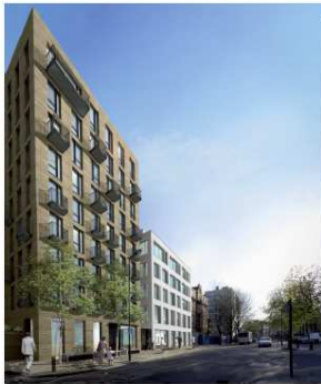
Unison HQ, Residential, Camden
