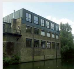
Camden Canal Side Architecture
