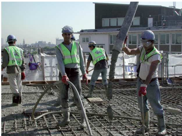
Sub-contractors at 199 Knightsbridge, London
