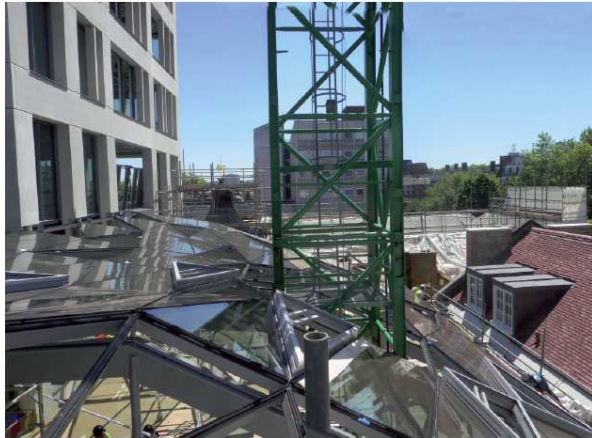
Unison Headquarters, Camden, London
