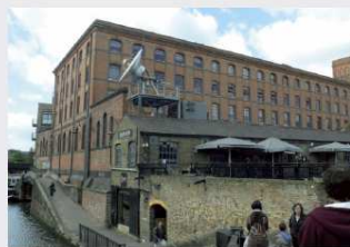
Camden Large Industrial Warehouse
