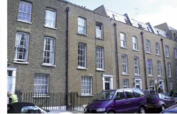
Typical Camden 19th Century Brick Terrace
