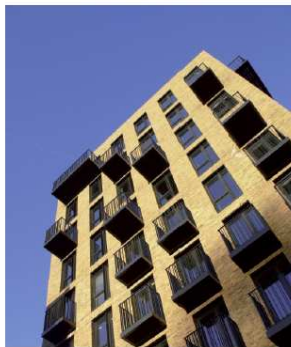
Unison HQ, Residential, Camden
