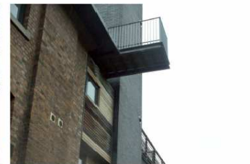
Typical Side Projecting Balconies
