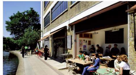
Canal Side Cafes at Bankstock Buildings.
