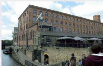
Camden Large Industrial Warehouse
