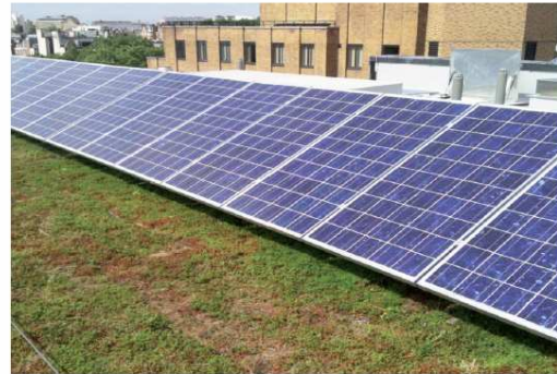
Green Roof and PVs at 1 Grafton Street, London.
