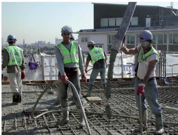
Sub-contractors at 199 Knightsbridge, London
