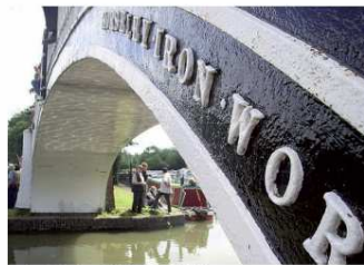
Typical Black and White Canal Bridge
