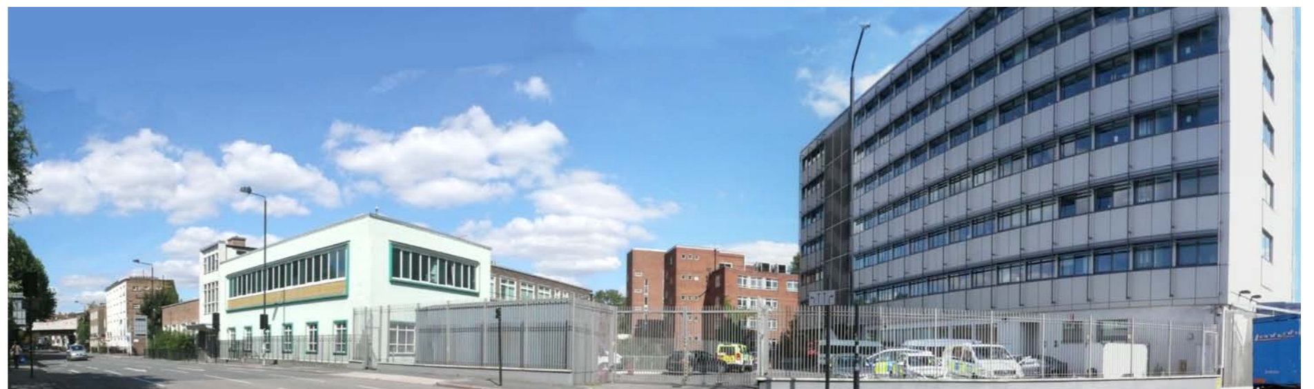
Fig 2.4.5 Buildings along Camden Street including Shirley House to the right occupied by the British Transport Police Offices
