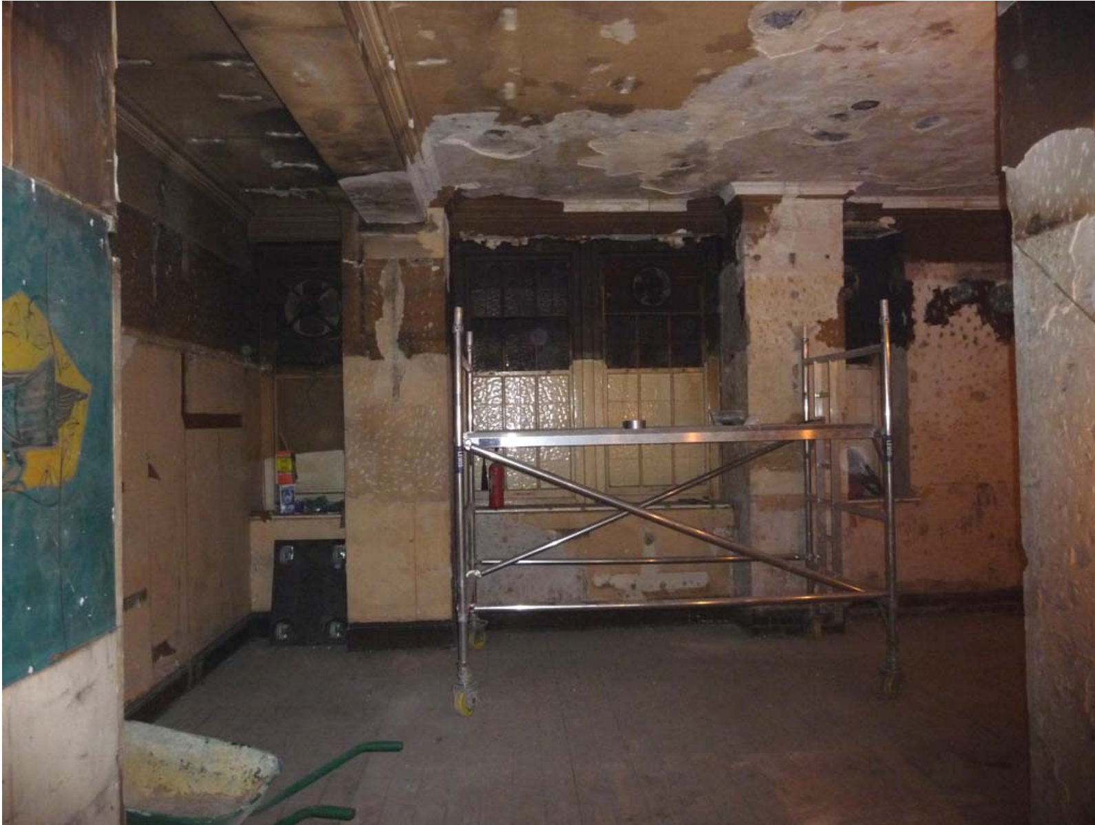
REAR WALL/BRICKED IN WINDOWS
