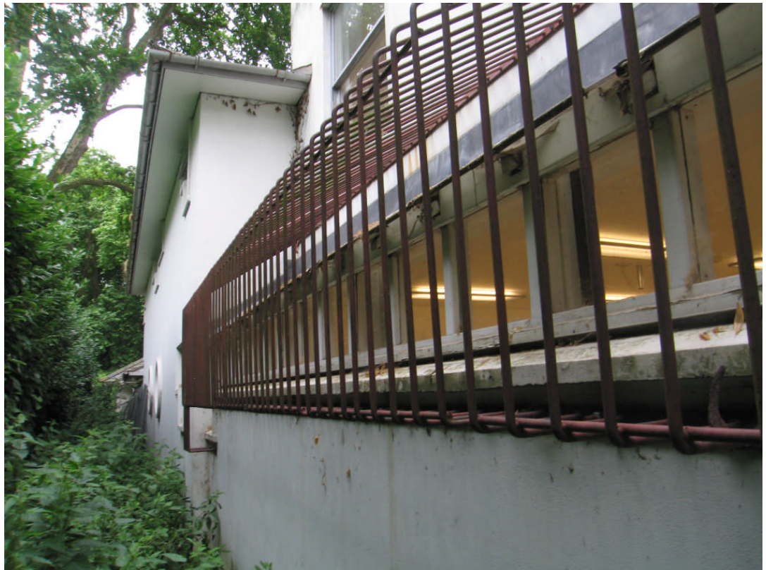
Photo 9: External view of existing timber lean- to & metal security bars.
