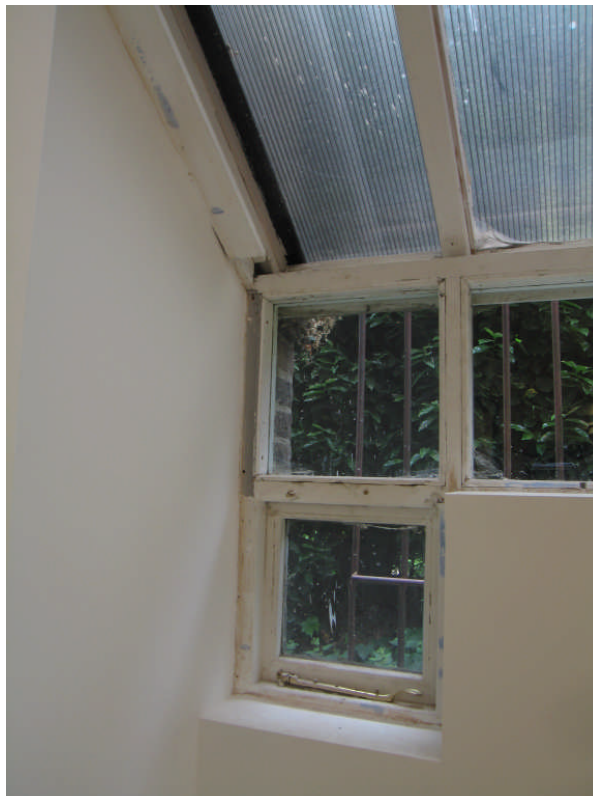
Photo 8: Internal view of existing timber lean- to & polycarbonate roofing.
