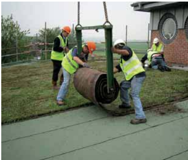
▲ Long length rolls being craned into position and installed.
