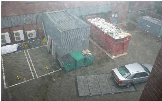
View of existing service yard, currently open to the elements
