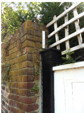
Poor quality repair with inappropriate brick stock
