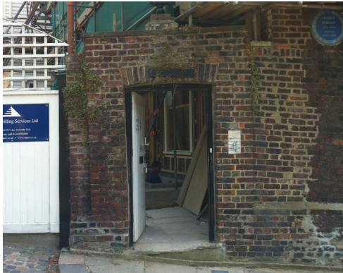
Inappropriate pointing
