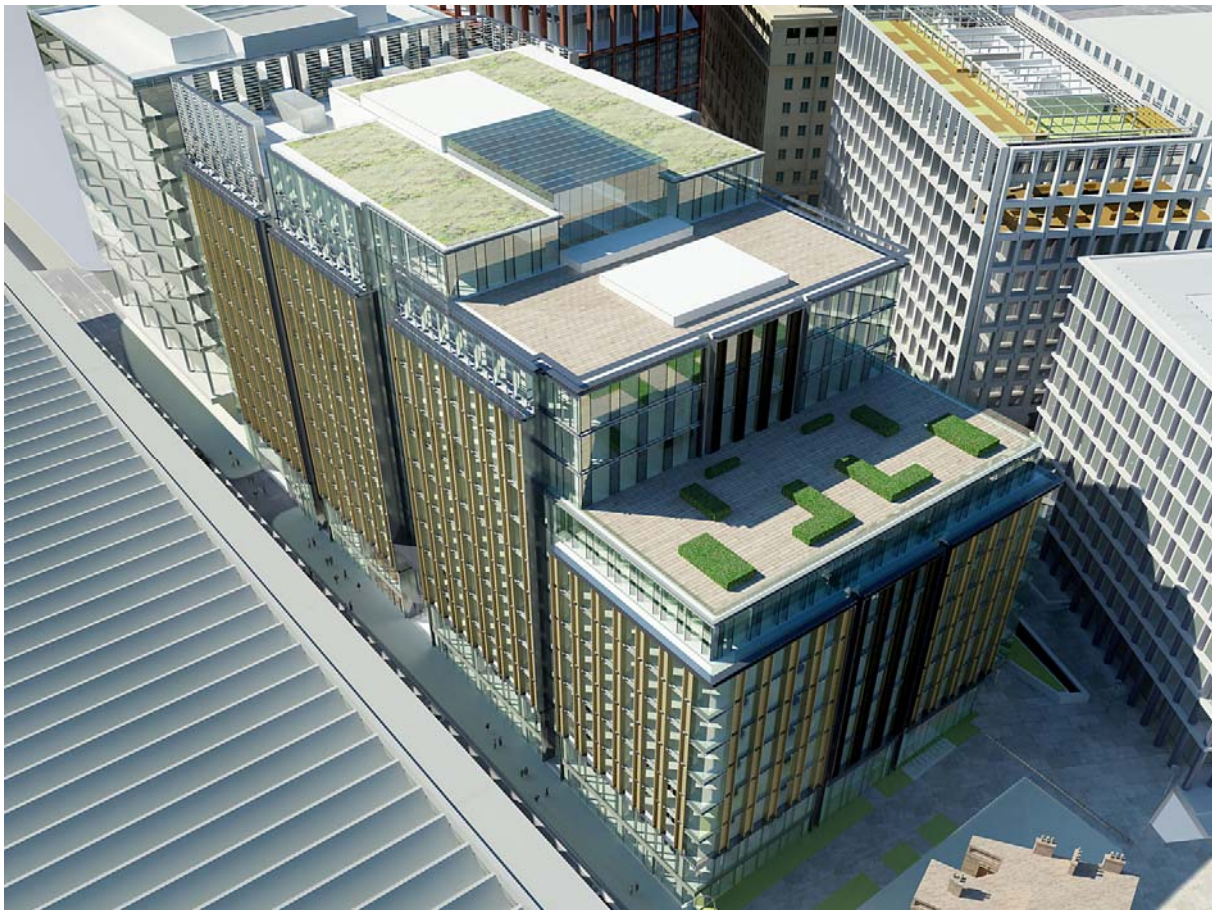
Figure 19: Building B1 - Visualisation of Roof level detail, showing brown roof area, terrace, atrium and landscape terraced levels.
