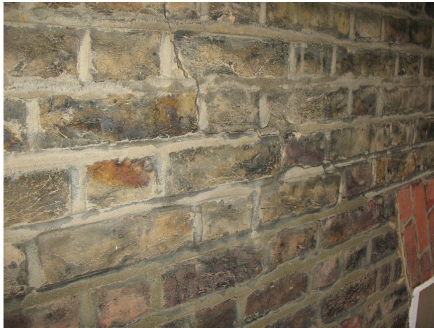
Photograph 3: Cracking to the rear of 17 Southampton Place
