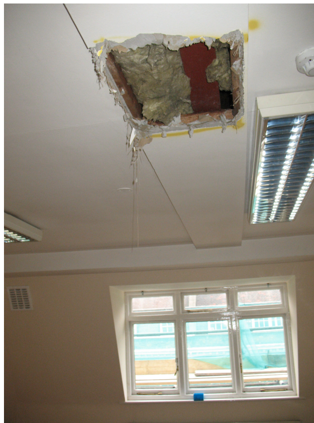
Photograph 2: Exposed steel roof beam in number 17
