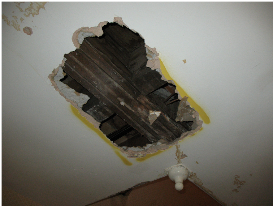
Photograph 4: Water ingress to the ceiling of 18 Southampton
