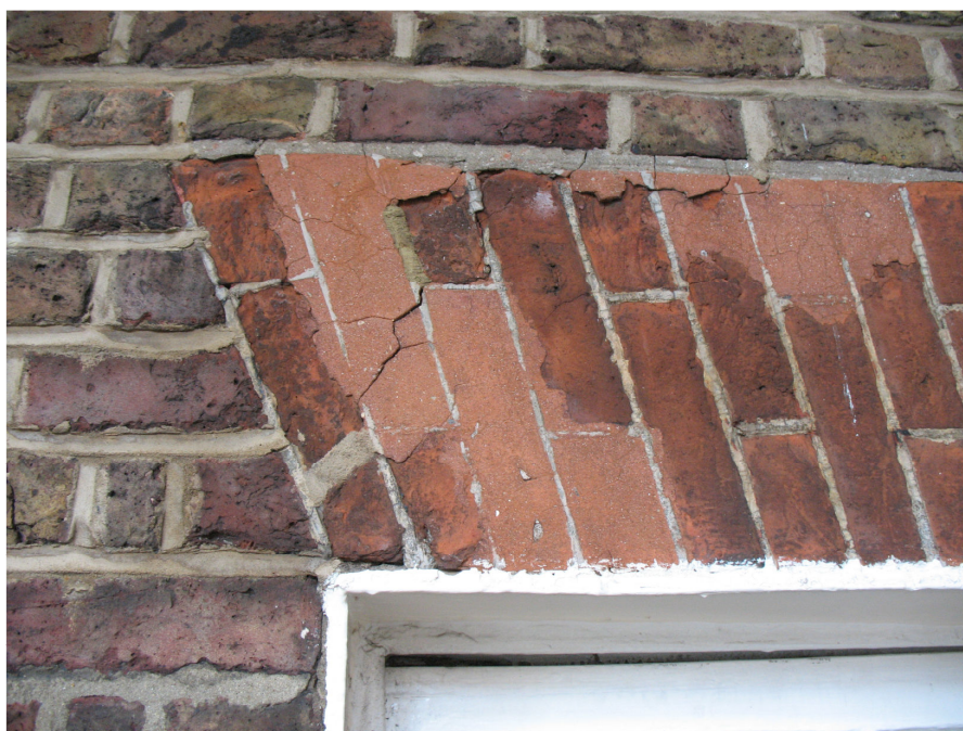
Photograph 5: Delaminating to the brick arch over the rear window of 18 Southampton Place.
