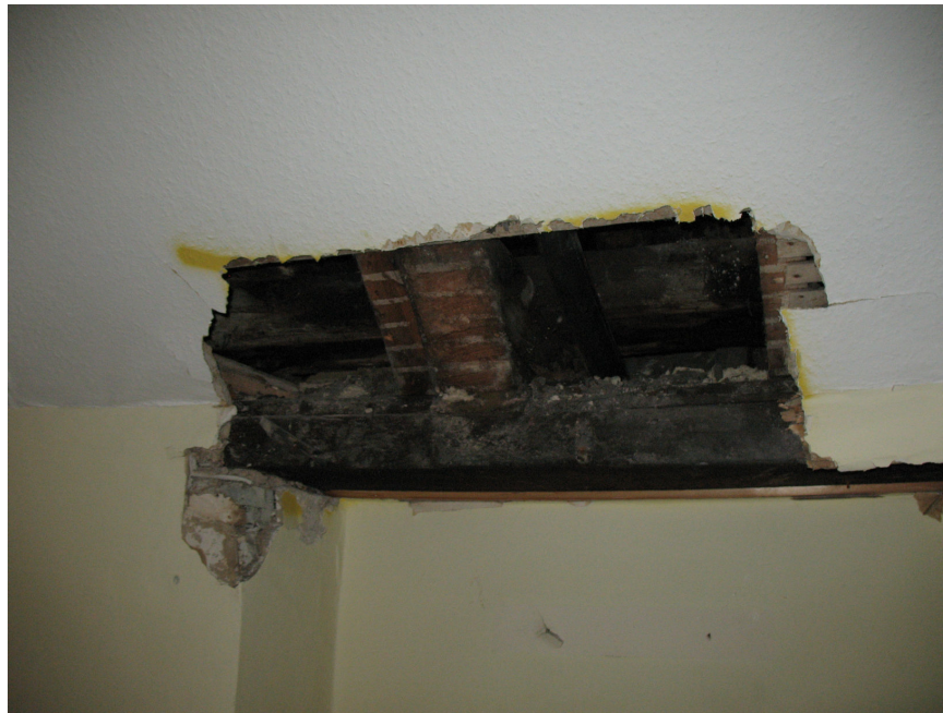
Photograph 1: Surface decay to valley of 16 Southampton Place
