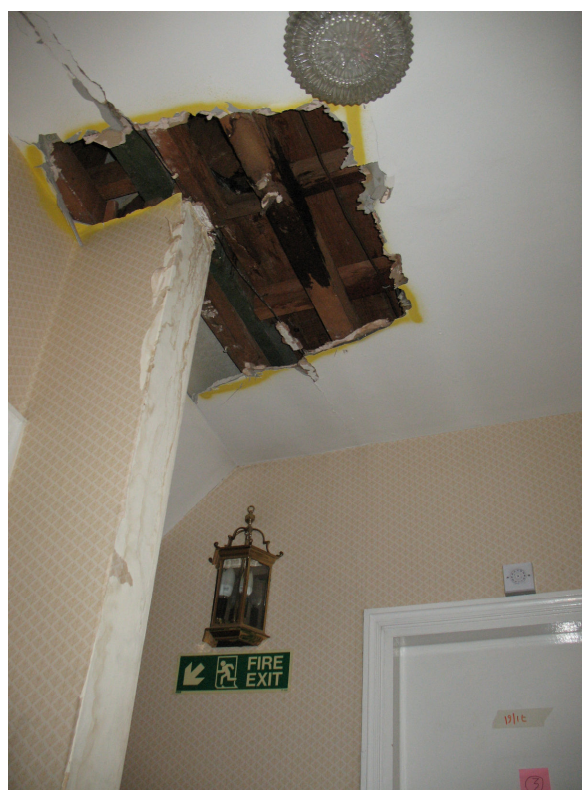
Photograph 6: Water ingress at third floor of 19 Southampton Place.
