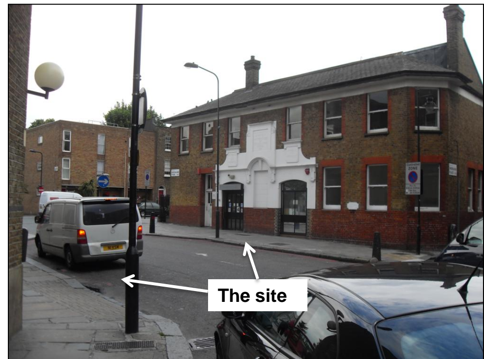
Figure 5.8: View of the site and the former Greenland Road Children's Centre
