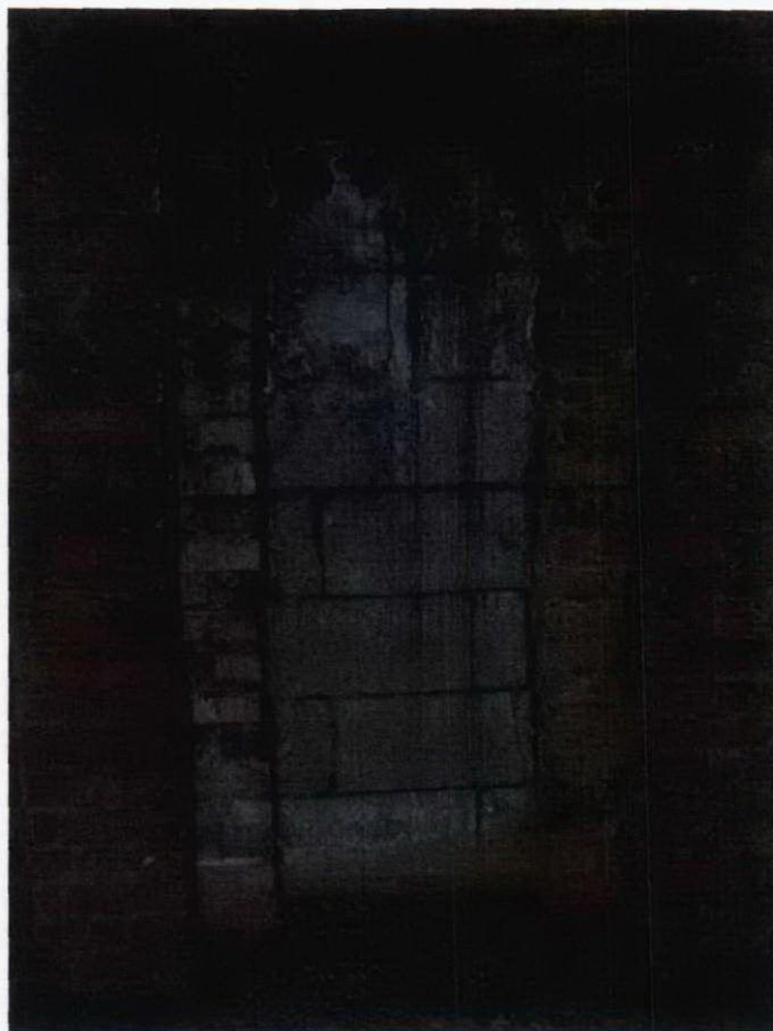
3: Middle vault (Vault 2), infill to historic opening to the original area, which will be temporarily removed in order to undertake the repairs.
