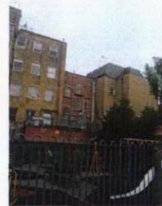
07 SITE PHOTOGRAPH REAR OF PROPERTY
