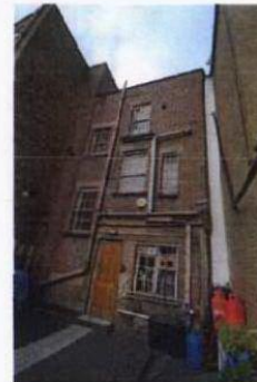
06 SITE PHOTOGRAPH REAR OF PROPERTY
