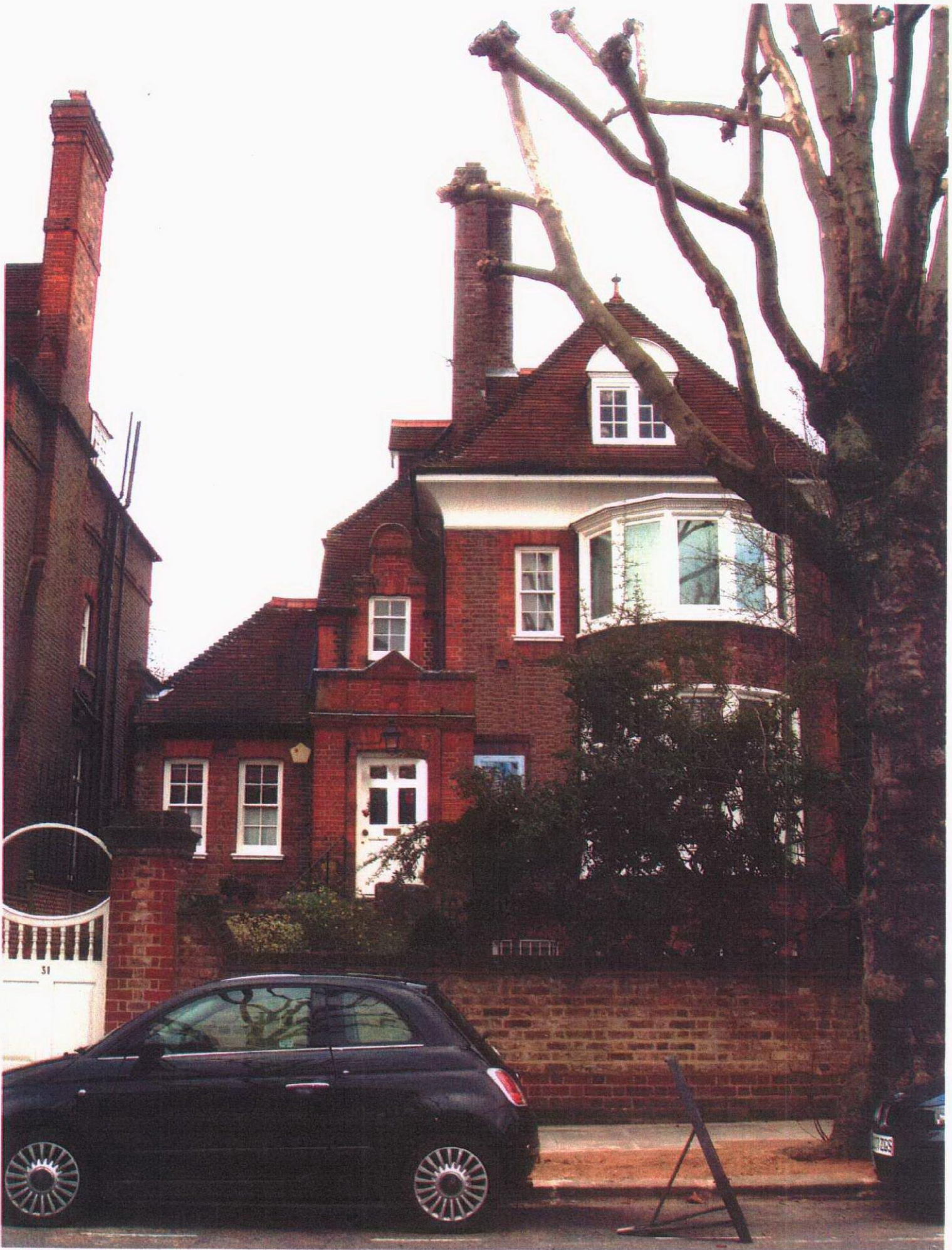
⑥ BUILDING PHOTO (AS AT PRESENT)
