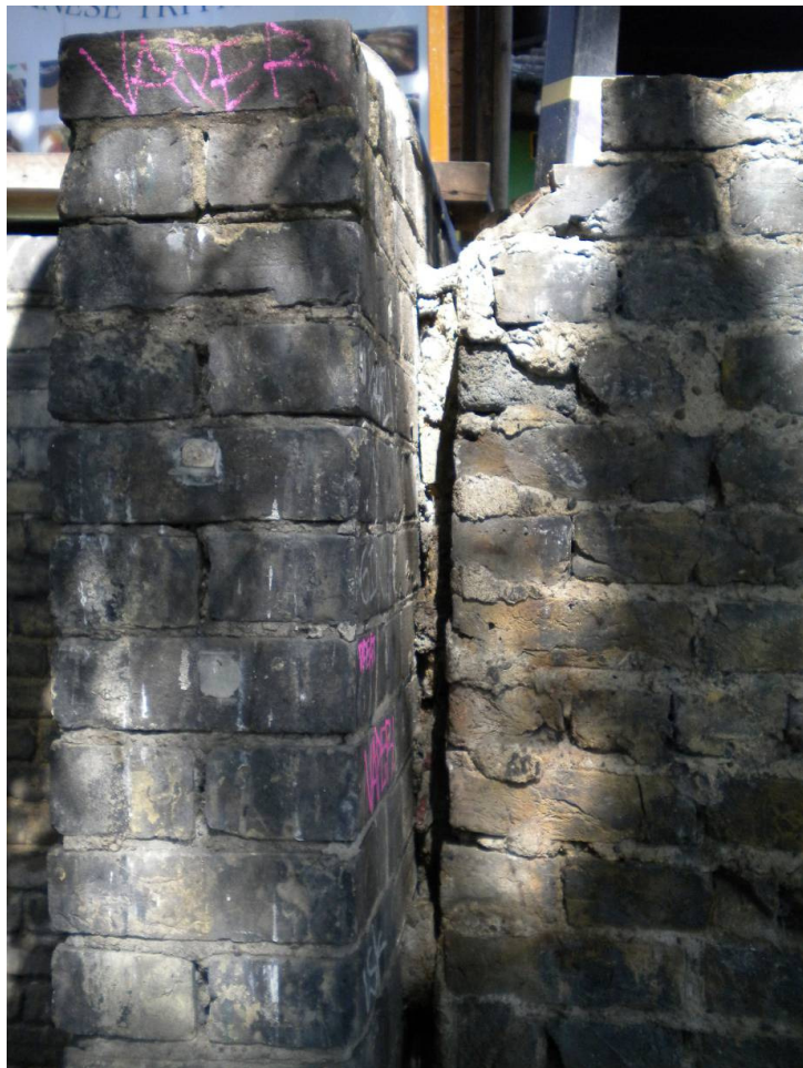
Fig. 12 Detail of the later parapet joining the end of the abutment.
