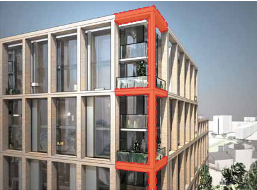
Removal of the brick frames enclosing the balconies
