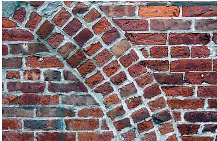
Arched brick lintel detail
