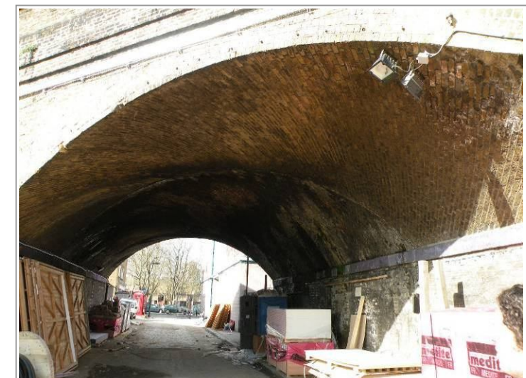
Fig. 17 Skewed brickwork arches within the subject site.
