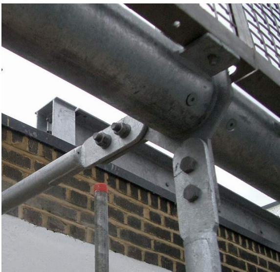
Galvanised Steel Hanger Connection Wimbledon Bridge, Wimbledon
