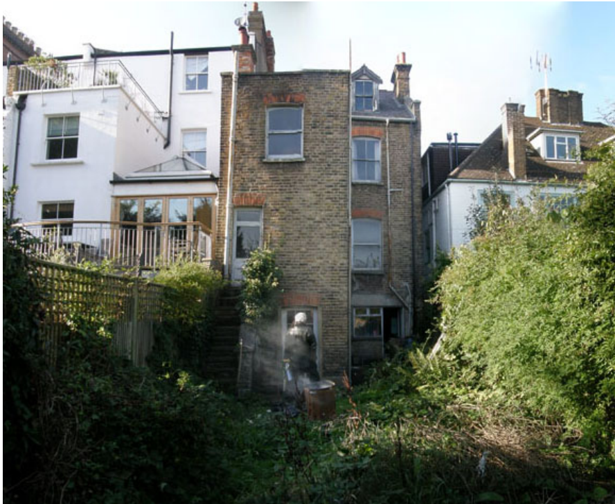
The Existing Rear Elevation
