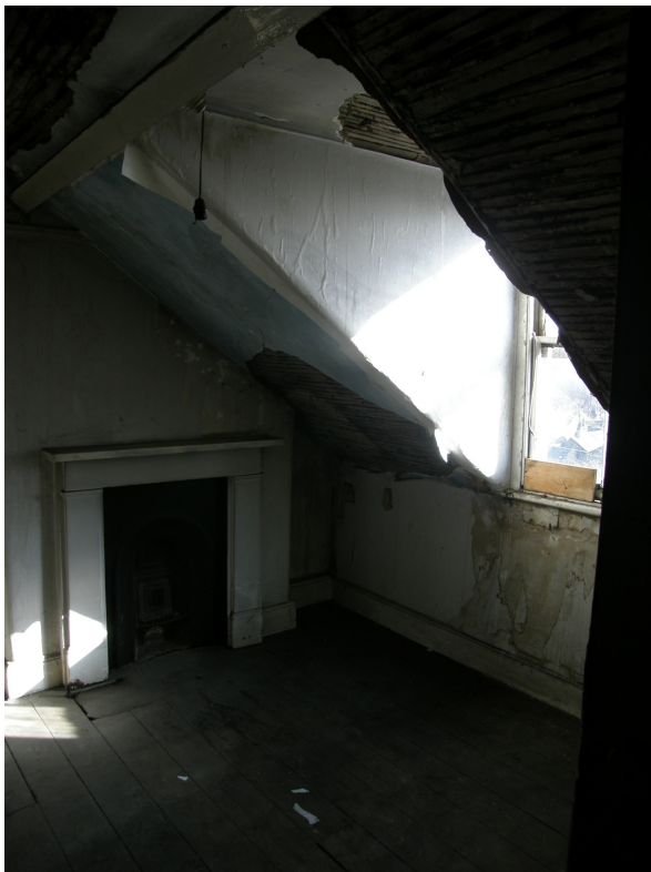
Existing Rear Dormer
