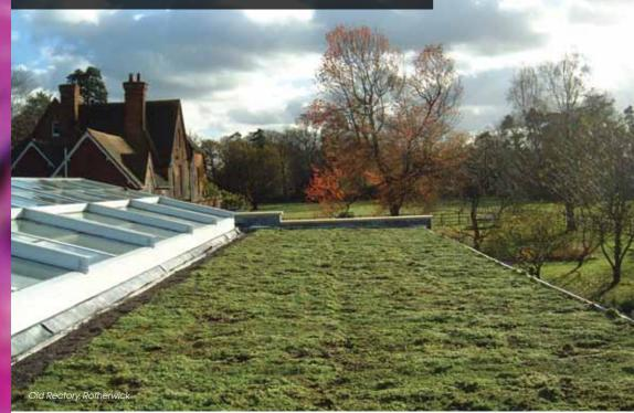
Lightweight extensive green roofs comprise a shallow layer of specially formulated growing media above filtration, drainage and waterproofing protection layers. The vegetation is selected from a range of drought tolerant plants including hardy succulents, grasses, herbaceous perennials, native wildflowers, alpines and bulbs.
